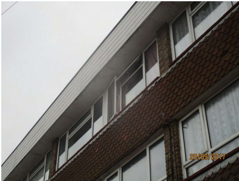
Photo 4 - Tile hanging to front elevation
