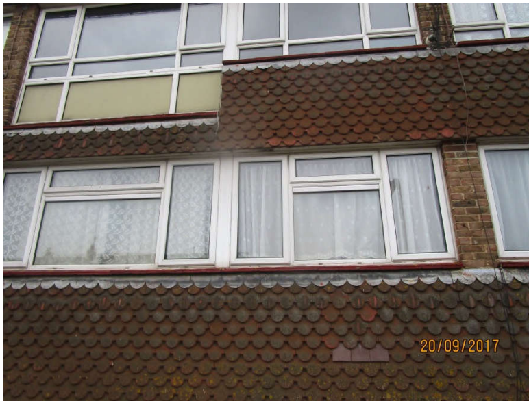
Photo 3 - Existing Fascia Board and Soffit
