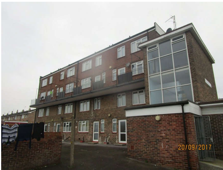
Photo 2 - Rear elevation showing balcony walkway
