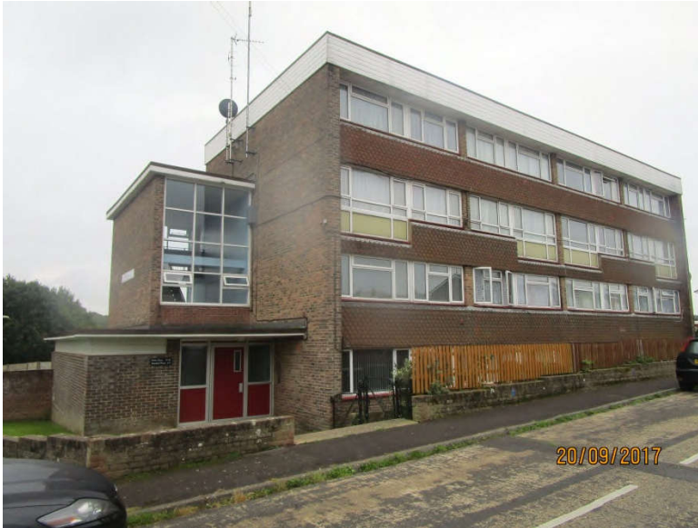
Photo 1 - Front Elevation showing boundary fencing
