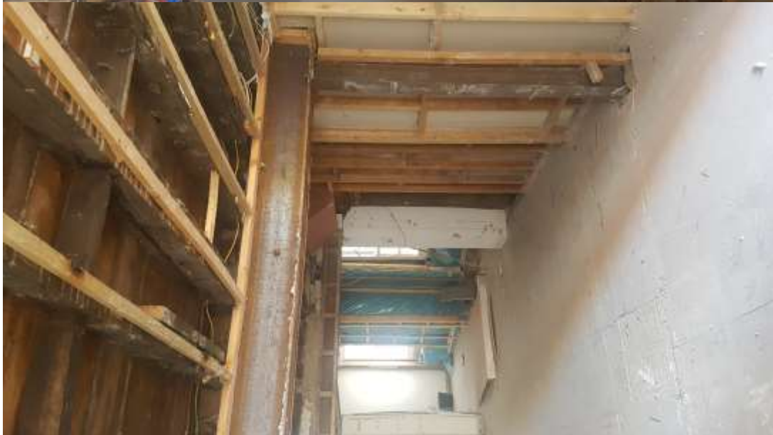
Steel frame continues into basement.
