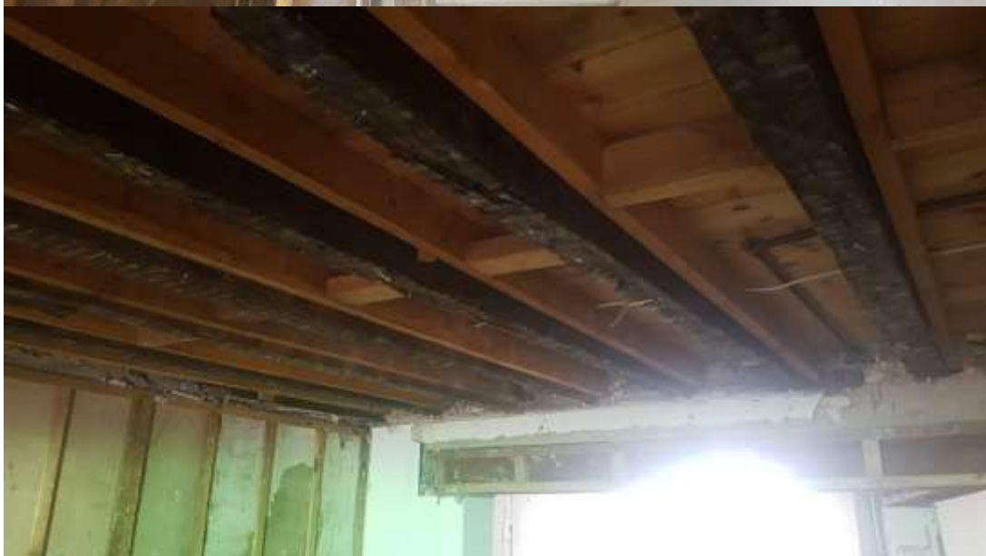
Double-joisted timbers have been installed due to structural integrity of existing timber joists.
