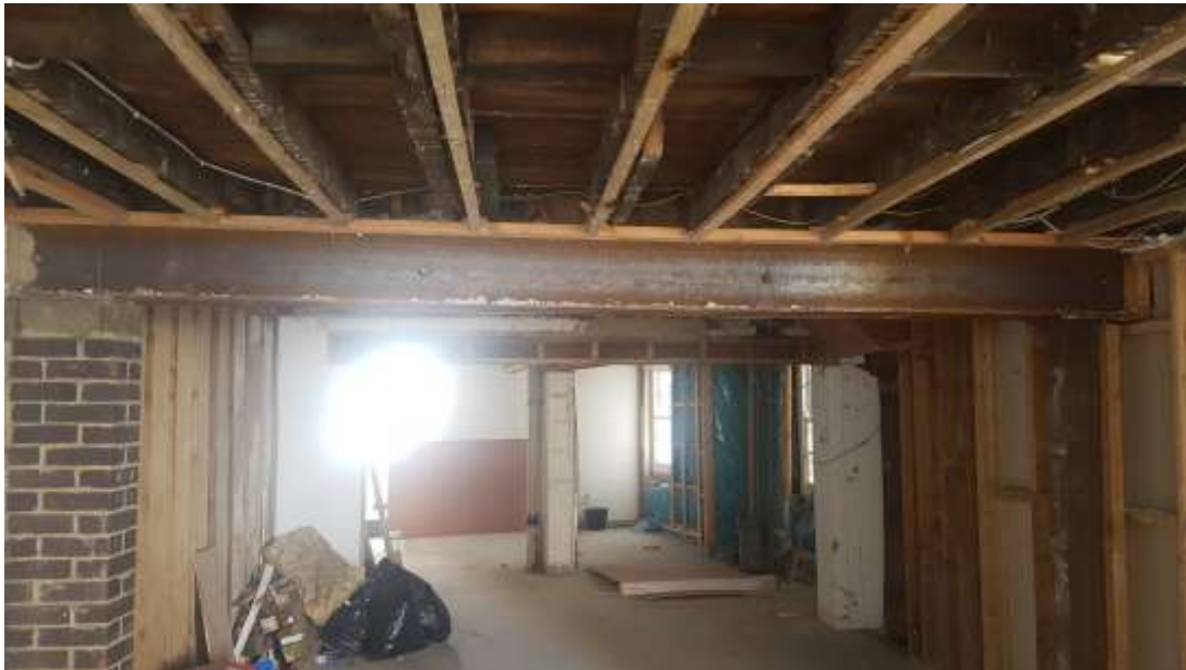
Interior back to front entrance showing existing steel frame and historic timbers in ceiling.
