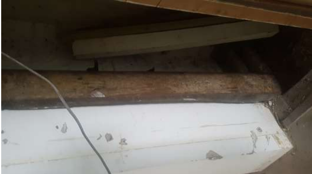
Historic timber upright at the top of the basement.
