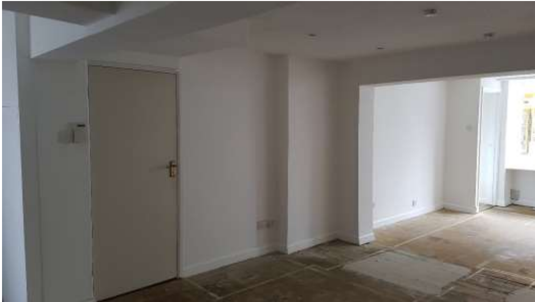
Interior back to front entrance showing door to basement prior to light demolition.
