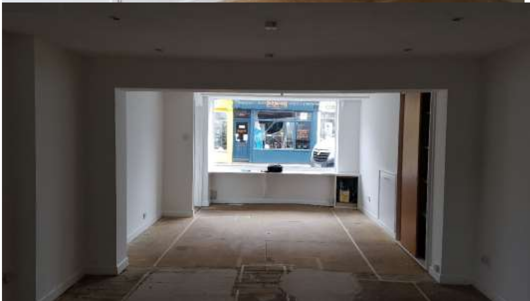
Internal view back to the main entrance prior to light demolition.
