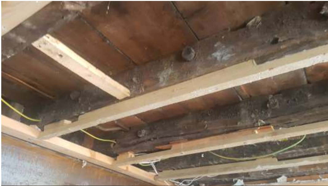
Historic timbers with timber pegs. Potentially reused timbers.
