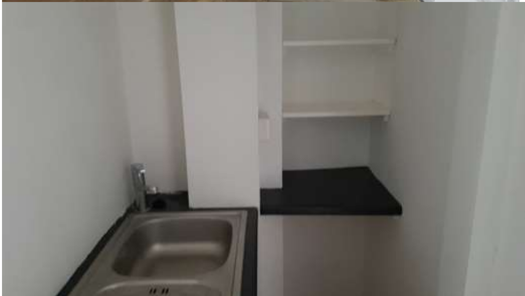
Internal kitchenette prior to light demolition.
