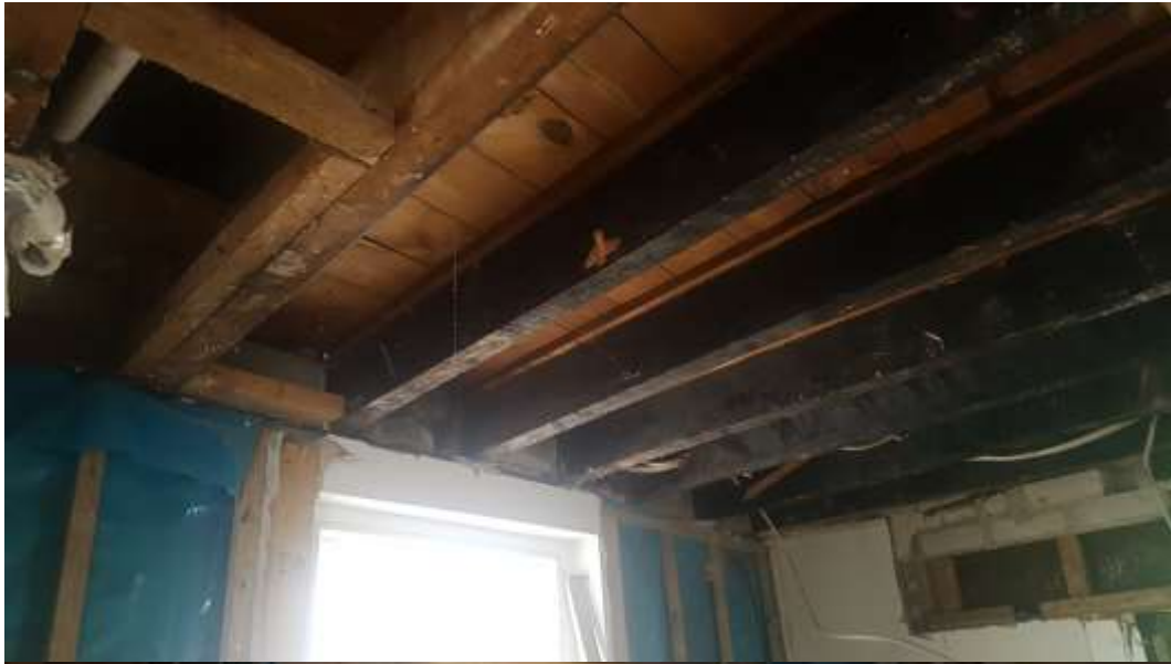
Historic timbers as part of two storey extension to the rear of the Georgian property.
