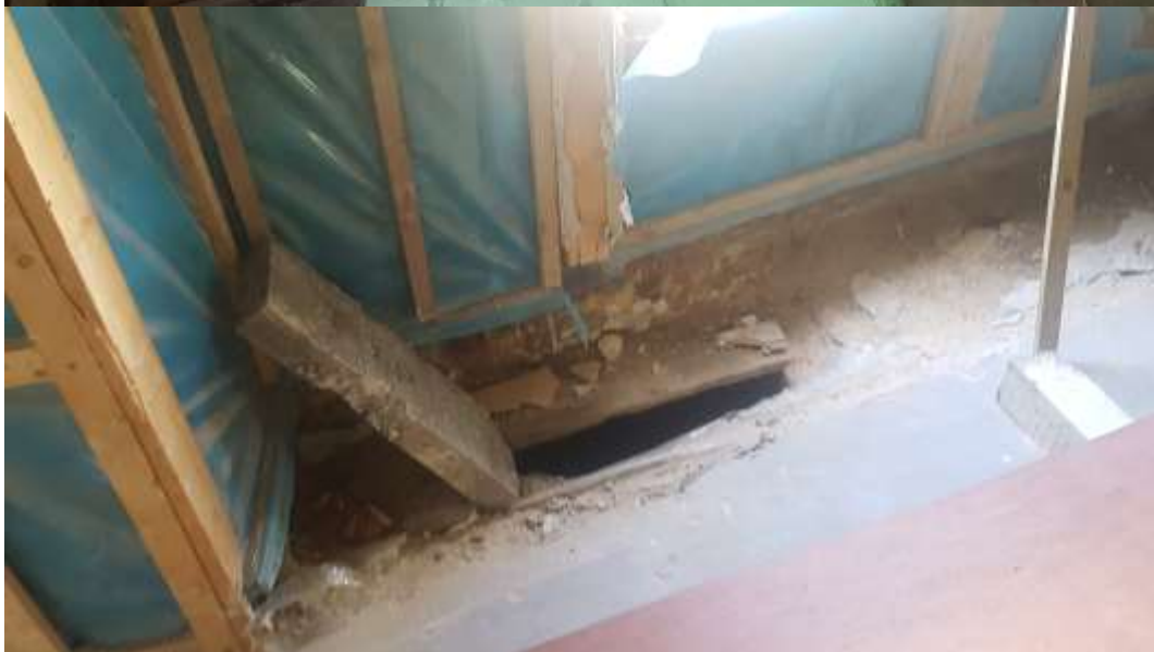
Top of well open with earth either side.
