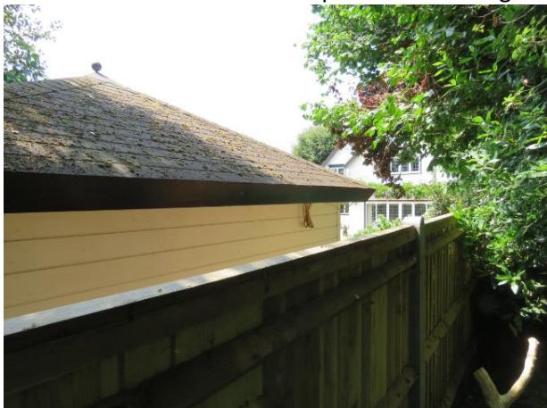
Photo of No. 3 Shawfield Road.
