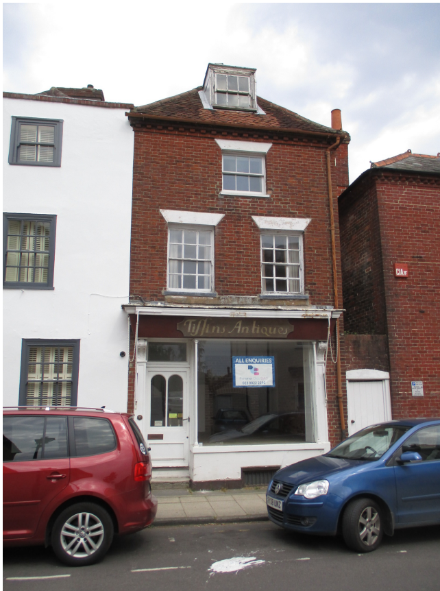
Fig 1 : View of street frontage of 12 Queen Street
