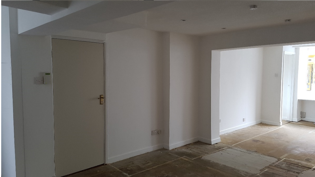
Interior back to front entrance showing door to basement.
