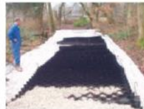
Installation of the CellWeb™ system.
