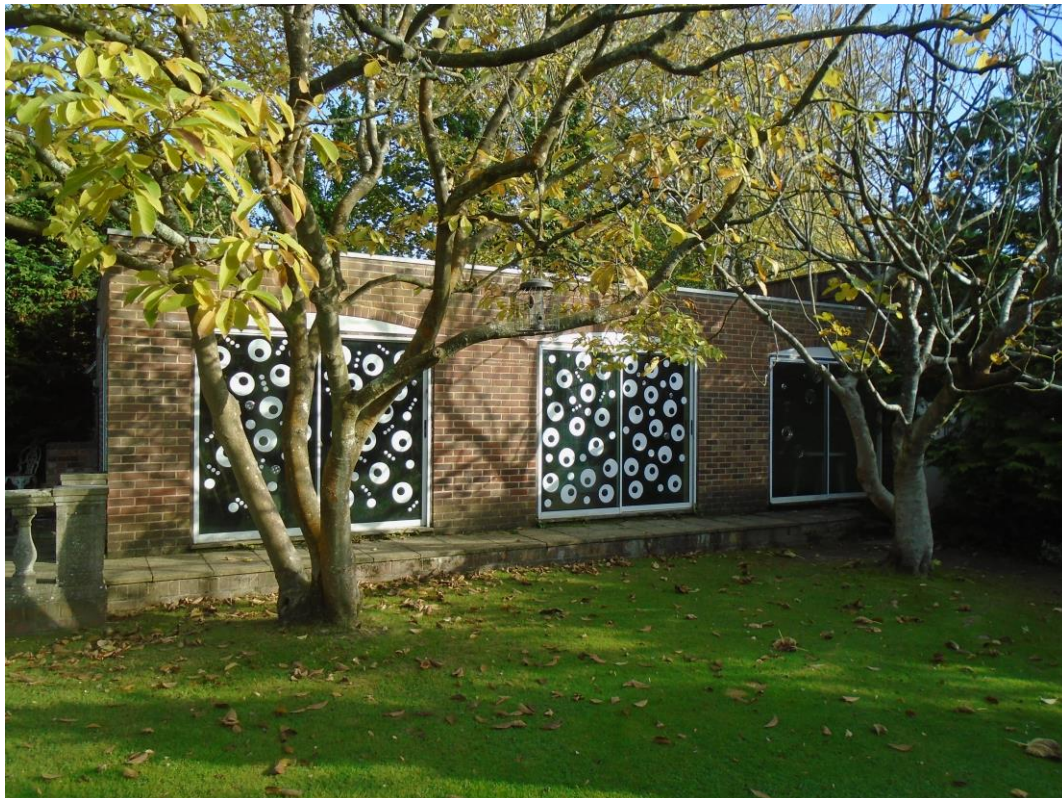
Figure 3. Unsympathetic design of pool house to be removed.
