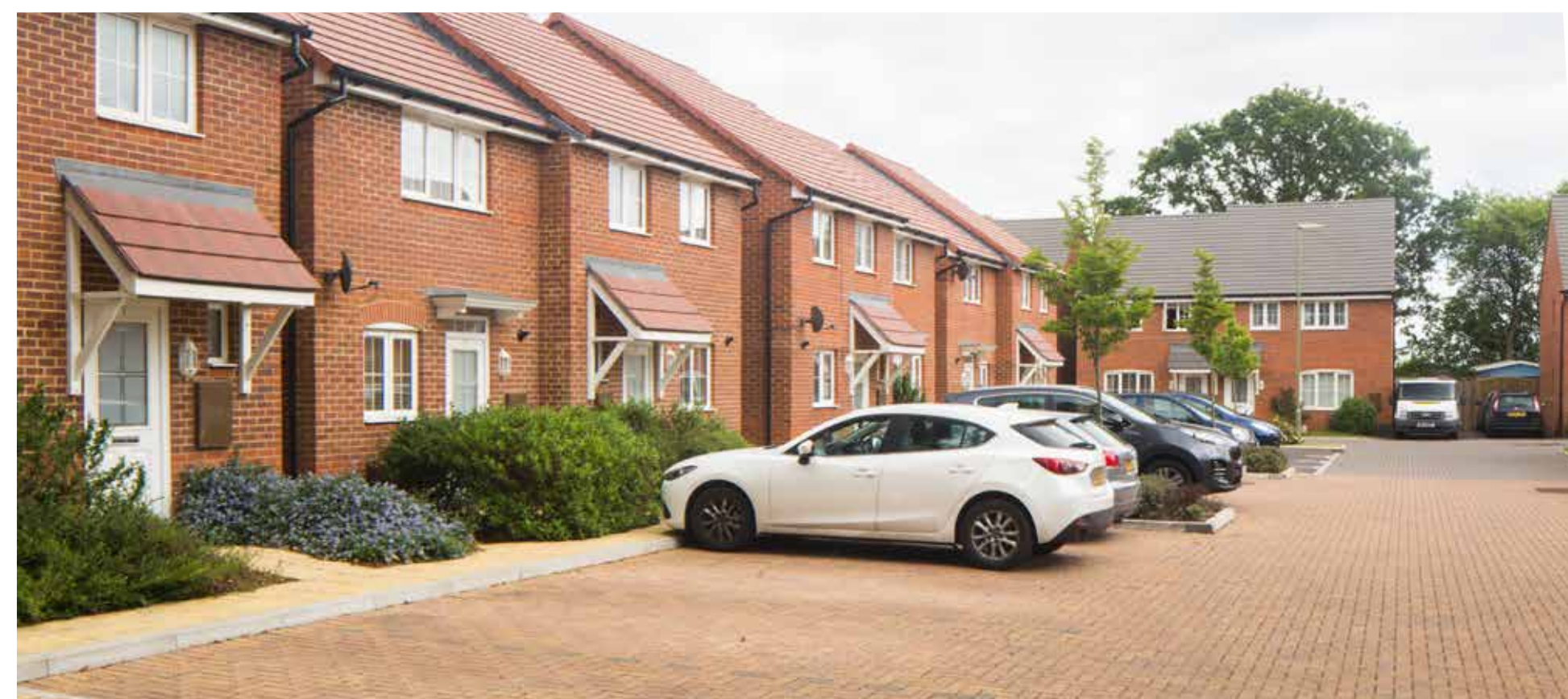
Examples of Permeable Paving Parking Bays
