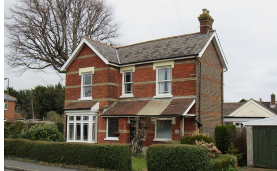
Red brick with contrasting buff brick bands, painted cills and lintels, sash windows and slate roof
