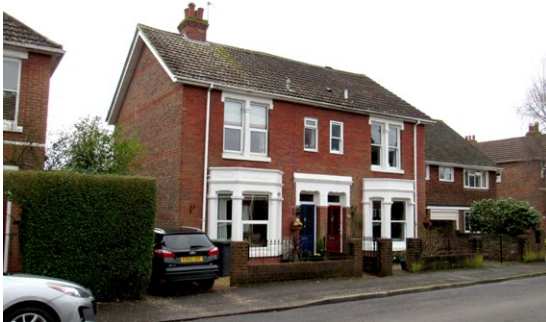
Red brick with concrete tile roof, painted bays, cills and lintels and sash windows
