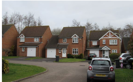
Azalea Close with landscape buffer to site behind
