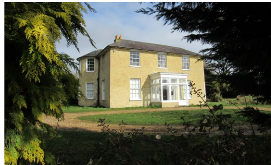
6. View of East Leigh House through northern boundary
