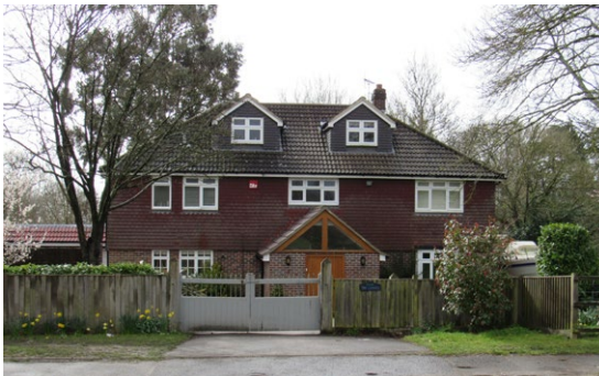
The Laurels directly adjacent to site access and backing onto northern boundary
