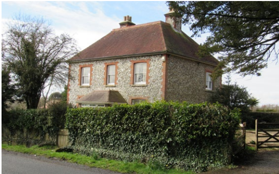
Cottage with Flint walls, red brick quoins and sash windows
