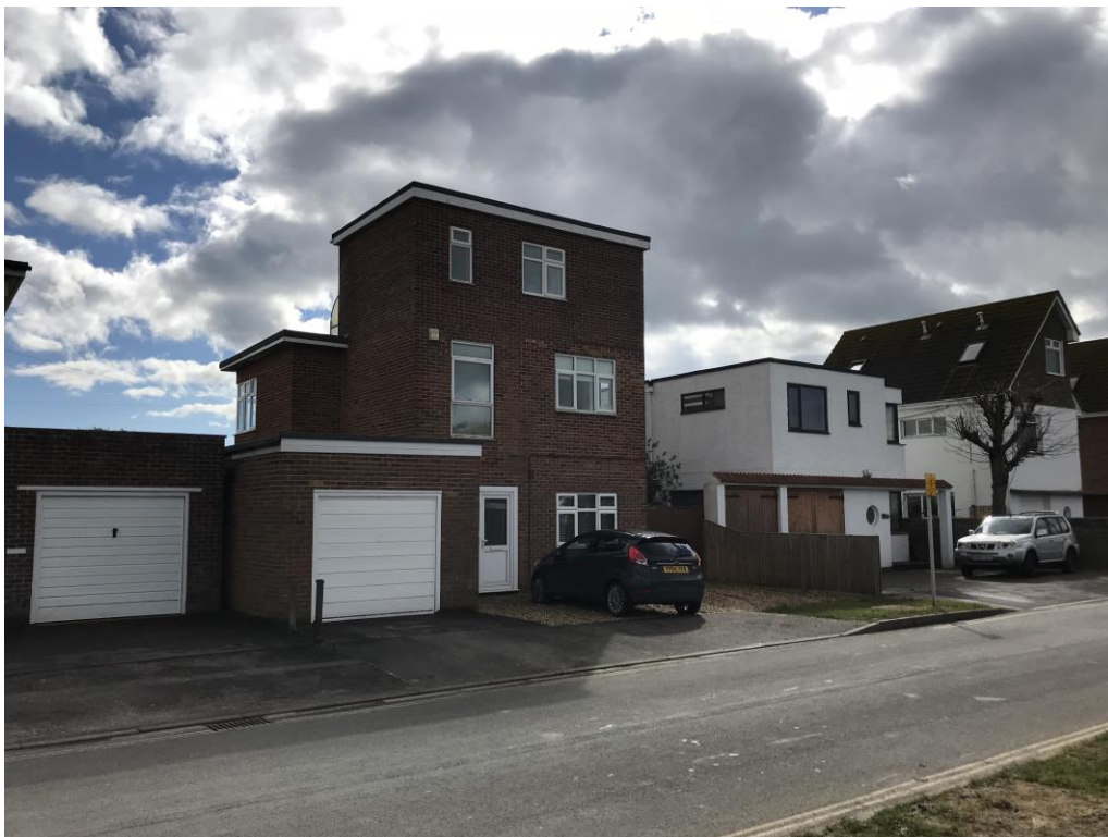
Figure 8: View down street comparing heights of application site (far left) and No 6 Bracklesham Road (far right)
