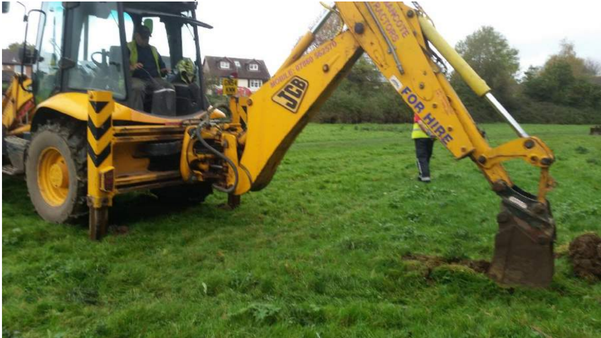
Photo 5: JCB used to excavate trial pits.
