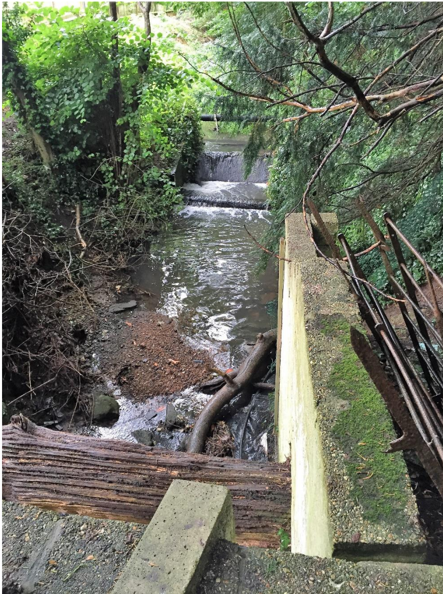
Figure 5. The beginning of the culvert at the northern end of the site that runs north to south underneath the site.
