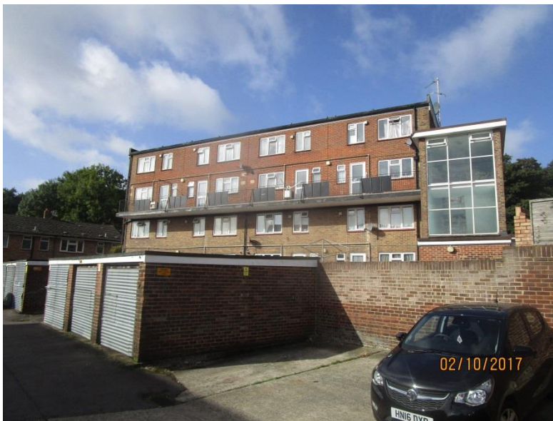
Photo 2 - Rear elevation showing balcony walkway
