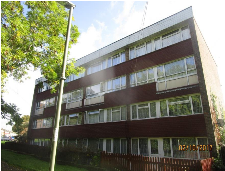
Photo 1 - Front Elevation showing boundary fencing
