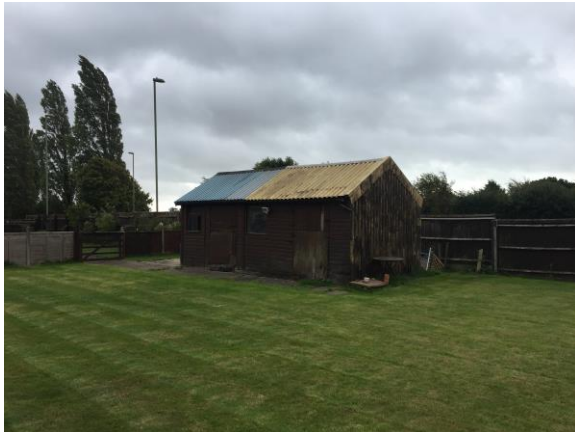
Figure 9/10: Existing outbuilding on south boundary
