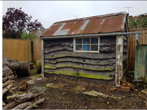
Photo showing the exterior of building B2
