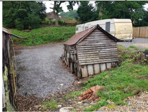
Photo showing the exterior of building B3
