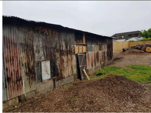
Photo showing the exterior of building B1
