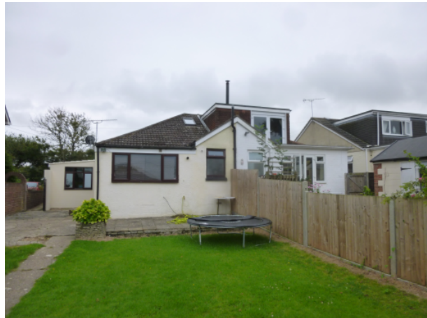
The rear elevations of nos.83 and 85 Geoffrey Avenue.
