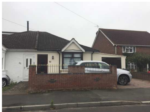
The application dwelling viewed from the east, on Geoffrey Avenue.
