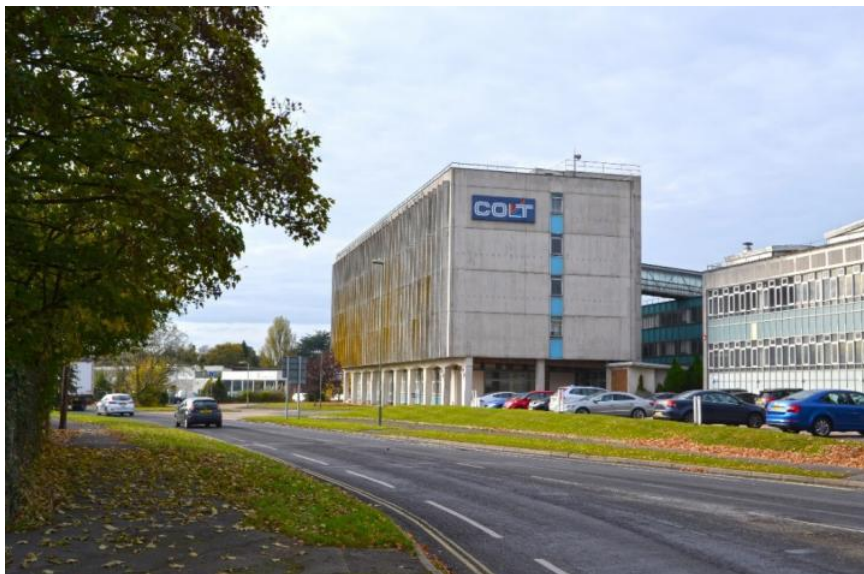
Figure 1: Former Colt International Building, New Lane, Havant
