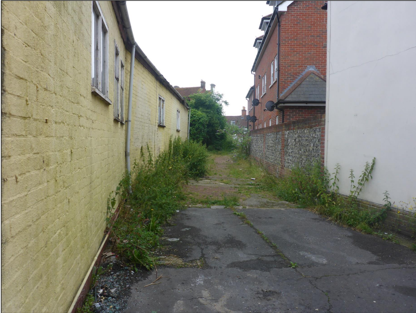
Figure 4. The access road to the rear
