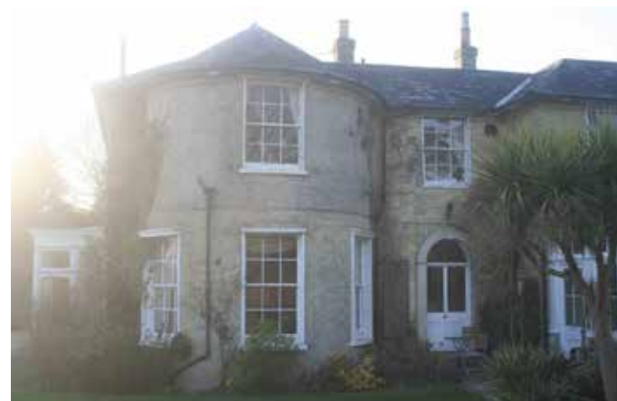
Above: View showing semi-circular bay to east elevation.
