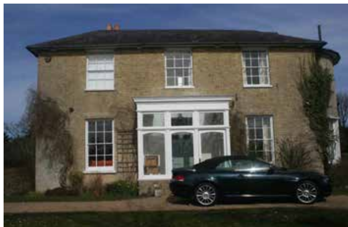
Above: South elevation of East Leigh House.
