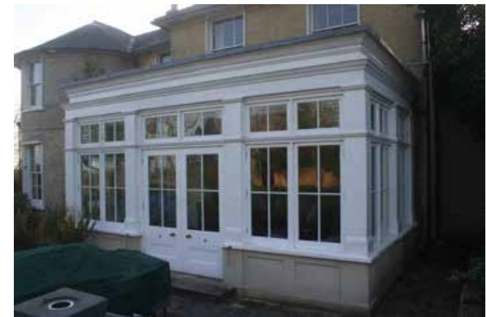
Above: The modern conservatory at the north-east corner of the building.
