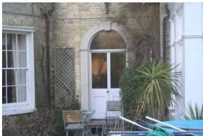
Above: Double door to east elevation of Regency building.
