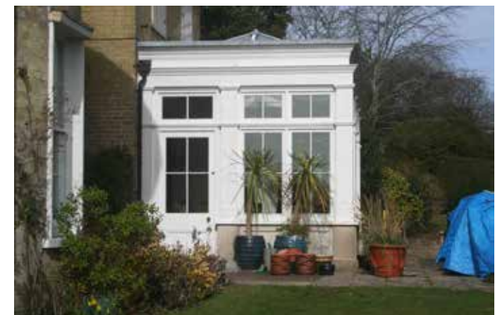
Above: South elevation of the modern conservatory.
