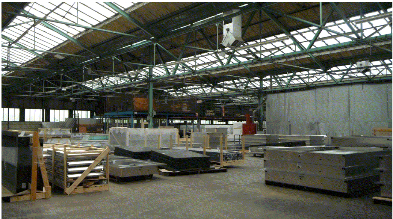
Photo 12 - View north west across southern portion of warehouse area
