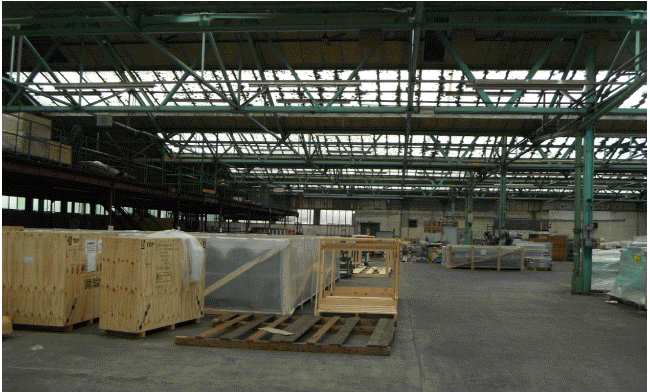
Photo 13- View north in western portion of warehouse
