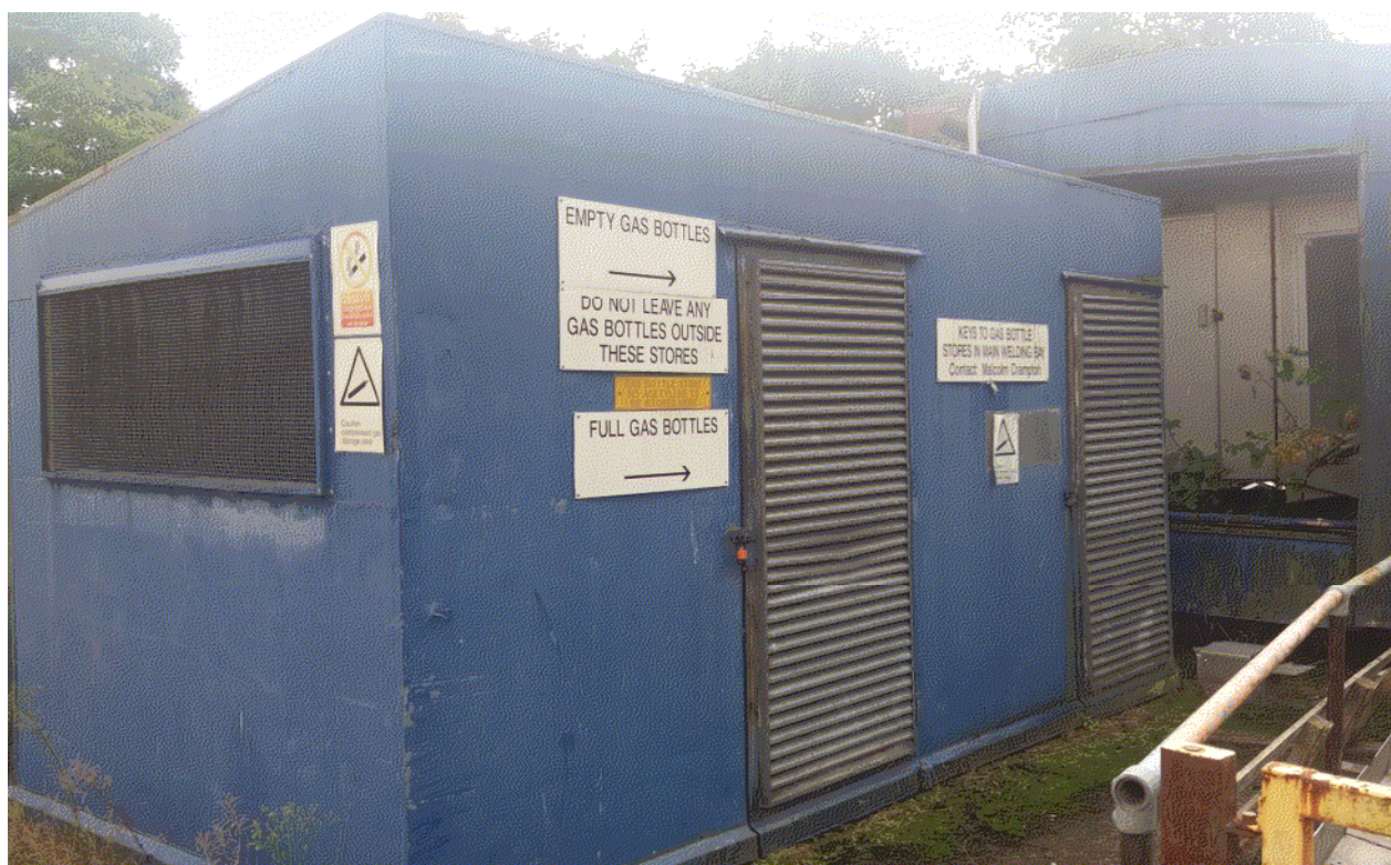
Photo 24 - External gas store in south of site
