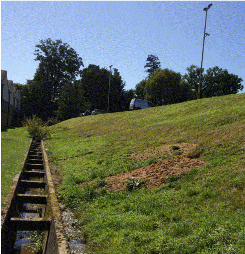
Photo 5 - View south along embankment and monsoon drain below the rear car park
