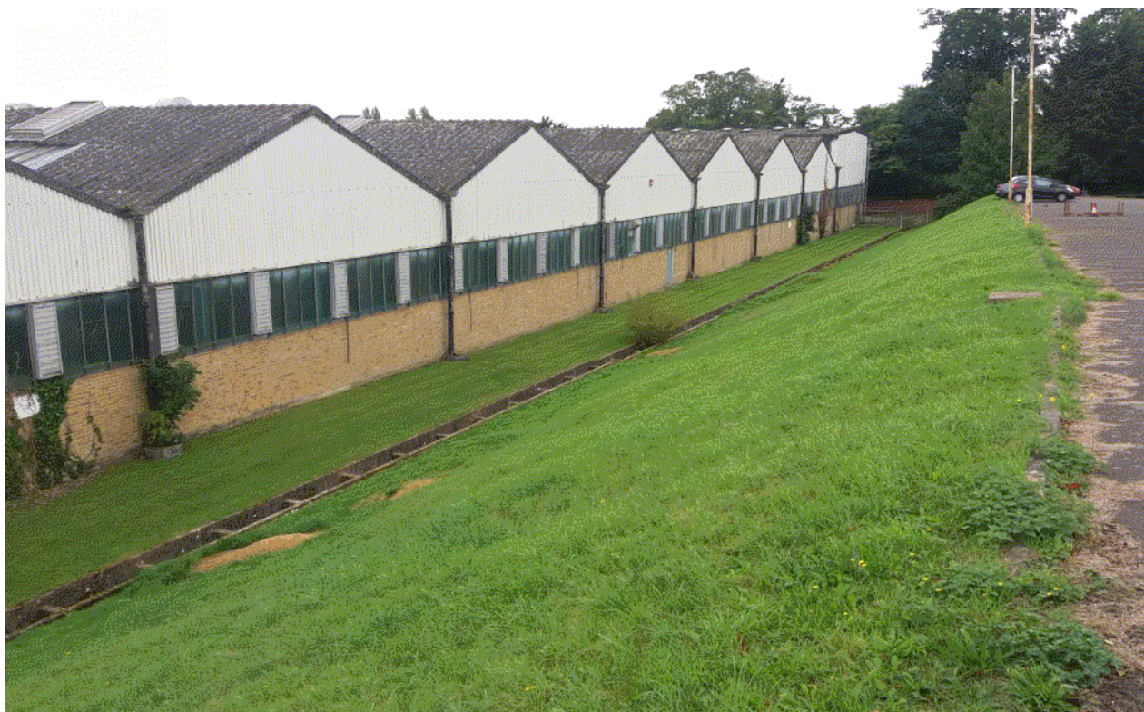
Photo 4 - View south along embankment and edge of rear (western) car park area
