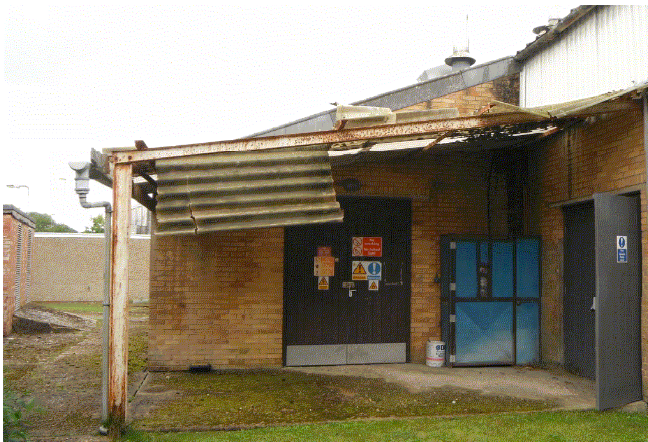
Photo 22 - Inaccessible building adjoining north edge of warehouse - identified as "Air pollution testing"
