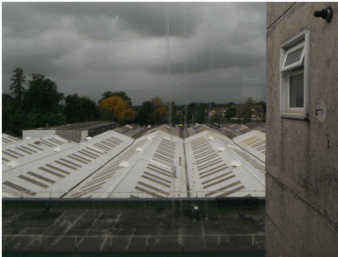
Photo 3 - View west from offices across factory and warehouse roofs
