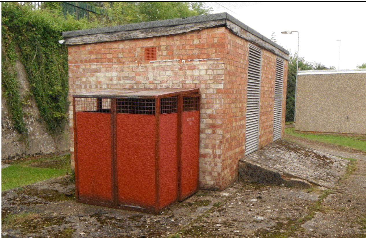
Photo 21 - Unidentified brick outhouse close to north site boundary
