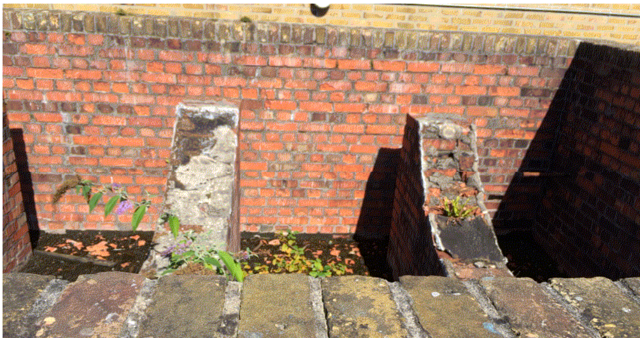
Photo 28 - Brick plinths inside bund of former diesel AST
