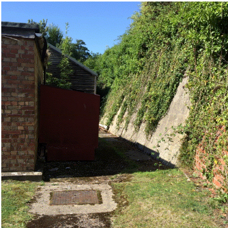
Photo 7 - View west along retaining wall at northern site boundary
