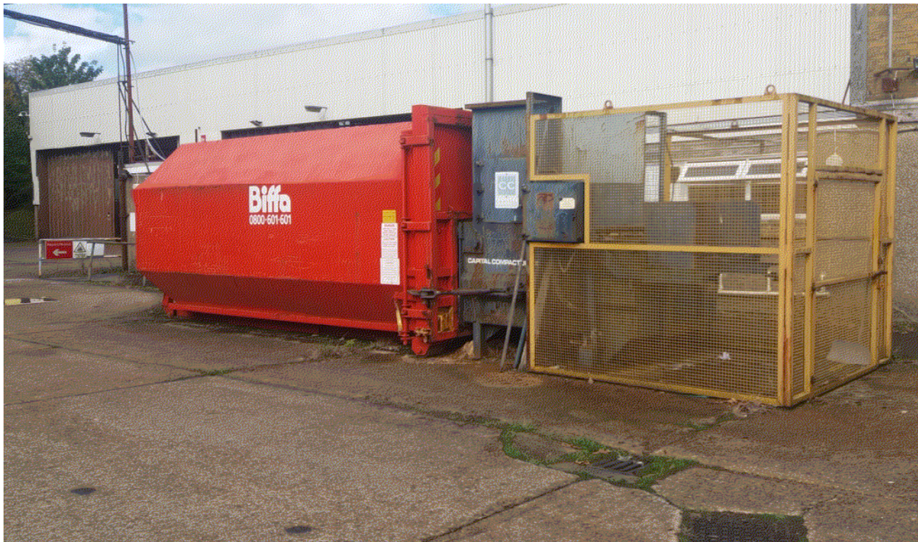
Photo 19 - Waste processing area to the south of factory building
