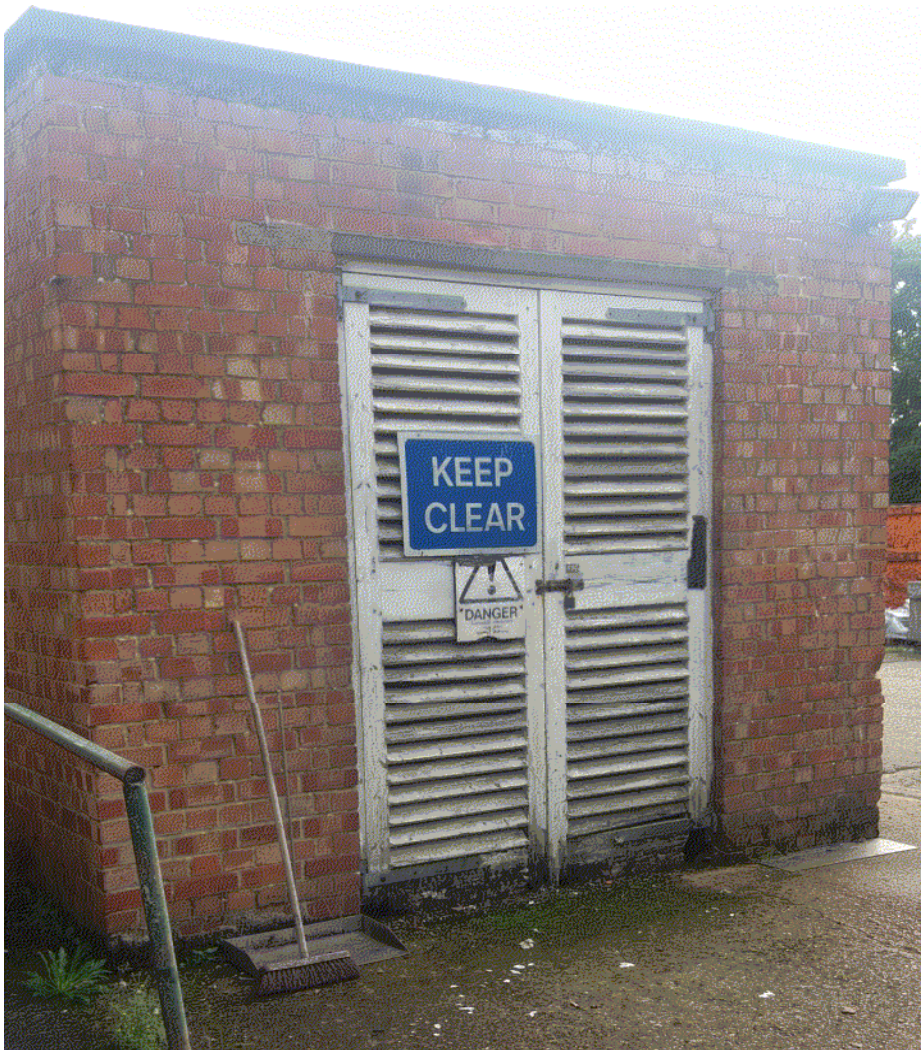
Photo 27 - Brick outhouse housing emergency generator
