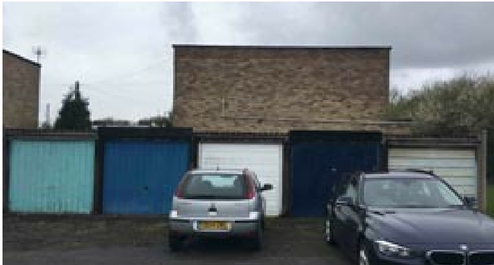
The single storey garages and flank elevation of the Juniper Square housing which occupies the majority of the West boundary.
