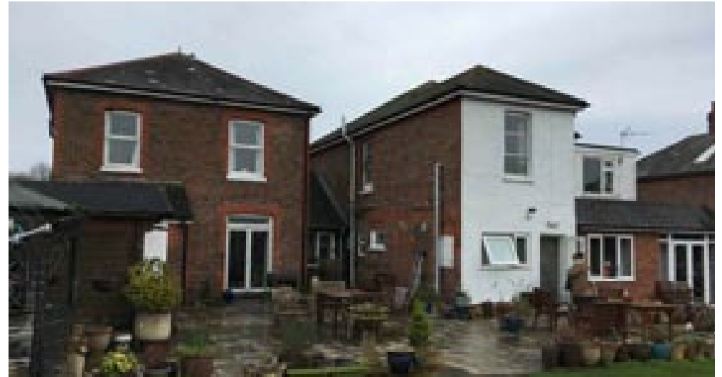
View of the rear of the buildings from the existing gardens
