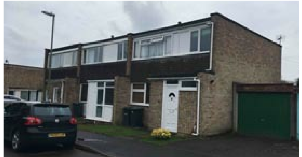
The existing housing looking towards the West boundary on Juniper Square.
