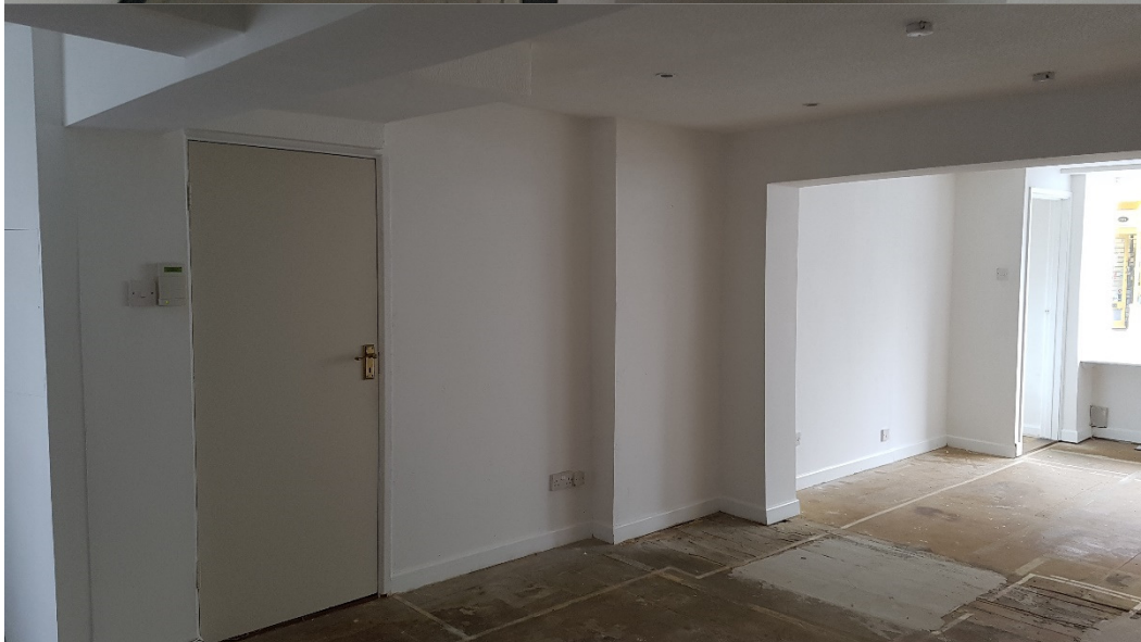
Interior back to front entrance showing door to basement.
