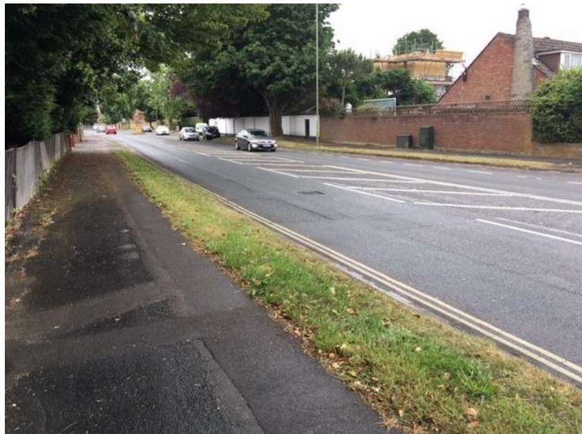
Photograph 2. Existing Pedestrian Infrastructure at Langstone Road.
