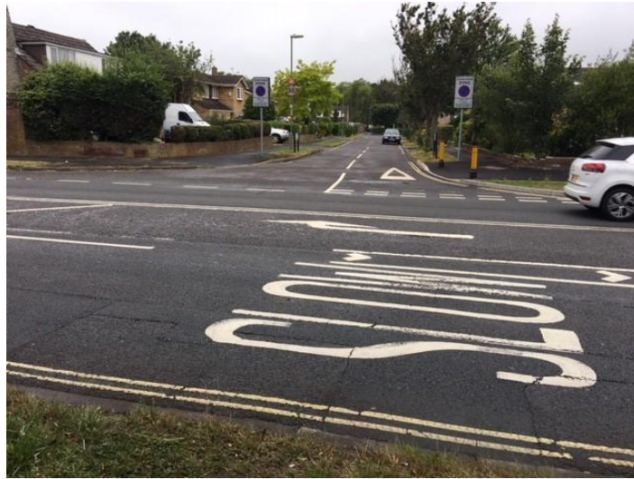
Photograph 7: Langstone Road/Langbrook Close Junction
