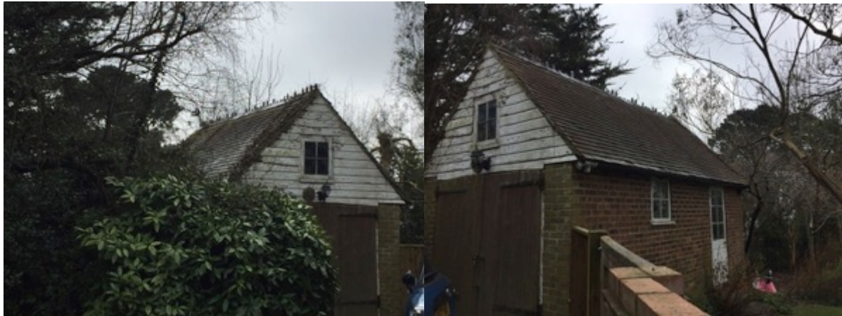
Figure 11. The garage within Plot 2 proposed for demolition. Left – North western and north-eastern faces. Right – North western and south-western faces.
