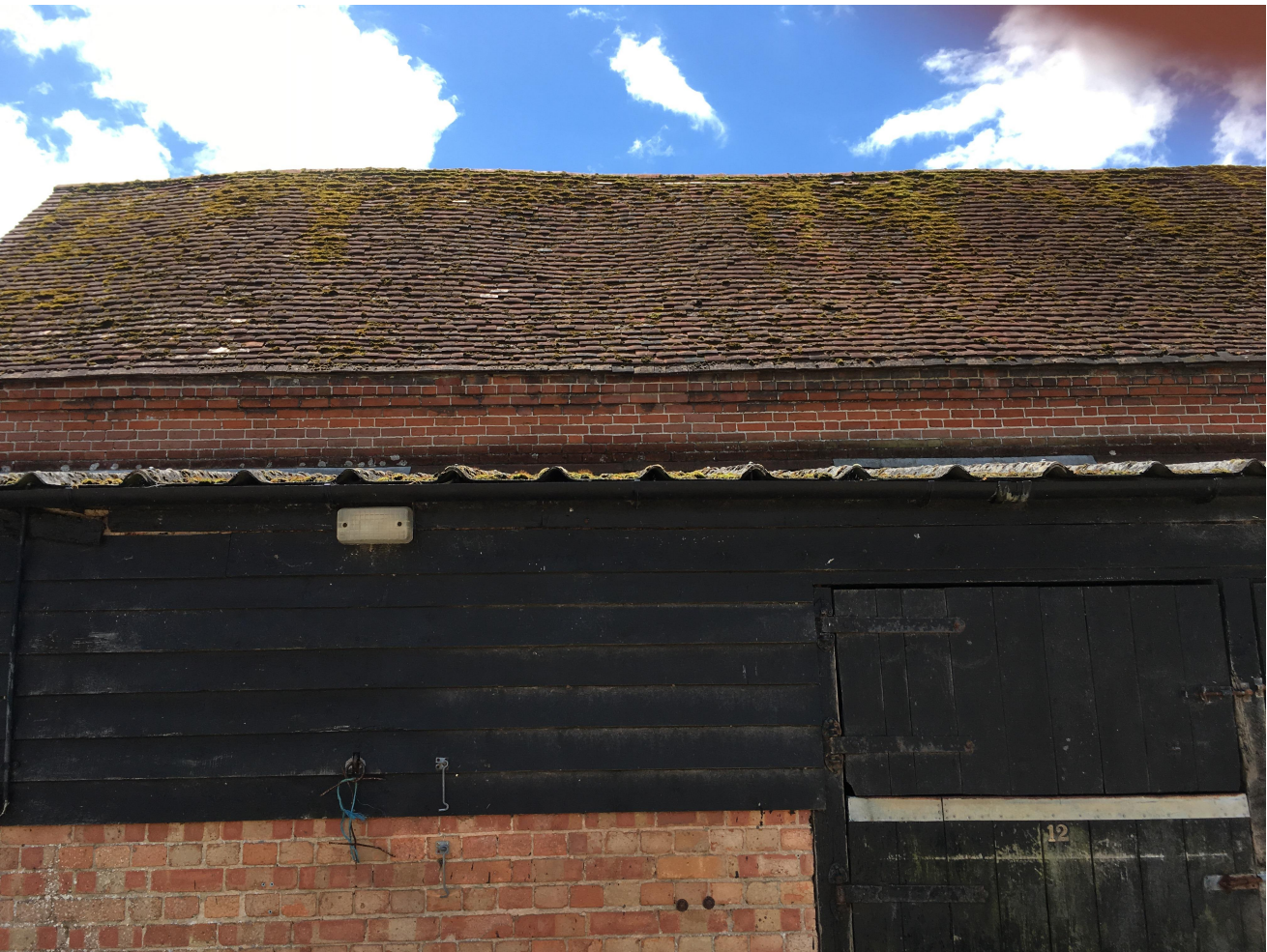
The existing clay tiled roof will be largely retained. A reclaimed equivalent wil extend onto the derelict east part of the stables.
