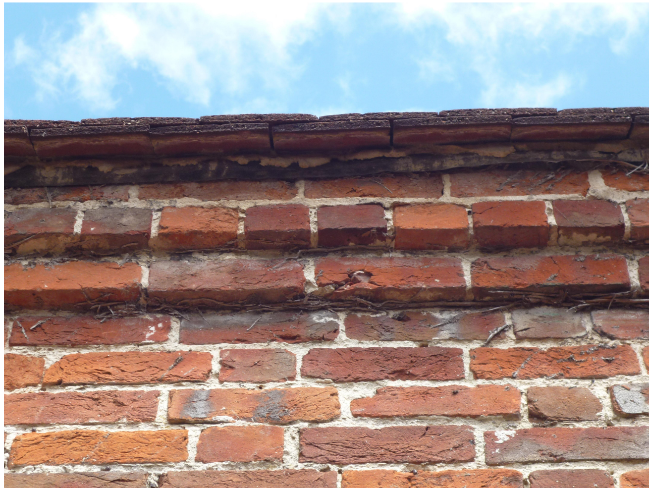
The existing brickwork will be repointed with soft lime mortar to match the existing. A large quantity of bricks arising from the ground will be re-used. Any new brickwork will be sourced from reclamation to match size colour and texture and will conform to the Sussex bond and occassional grey header as detailed within the Design, Access, Heritage and Planning Statement.
