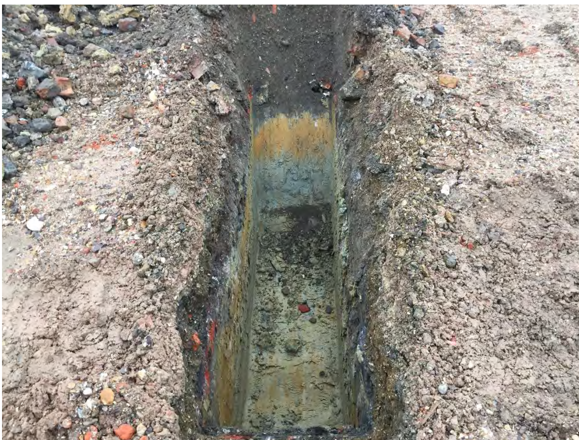
Photo 2: View within TP04. Note brick within Made Ground.
