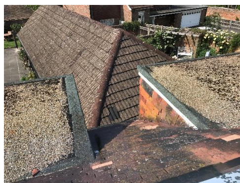
Existing first floor dormers and workshop roof.
