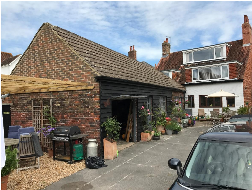
View of the barn (workshop) and rear elevation showing existing windows and dormers
