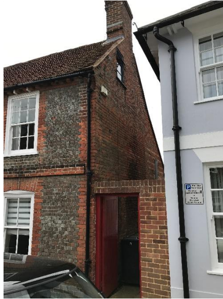
Archway and gate from King Street
