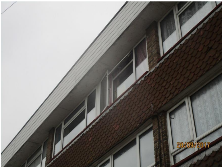
Photo 4 - Tile hanging to front elevation
