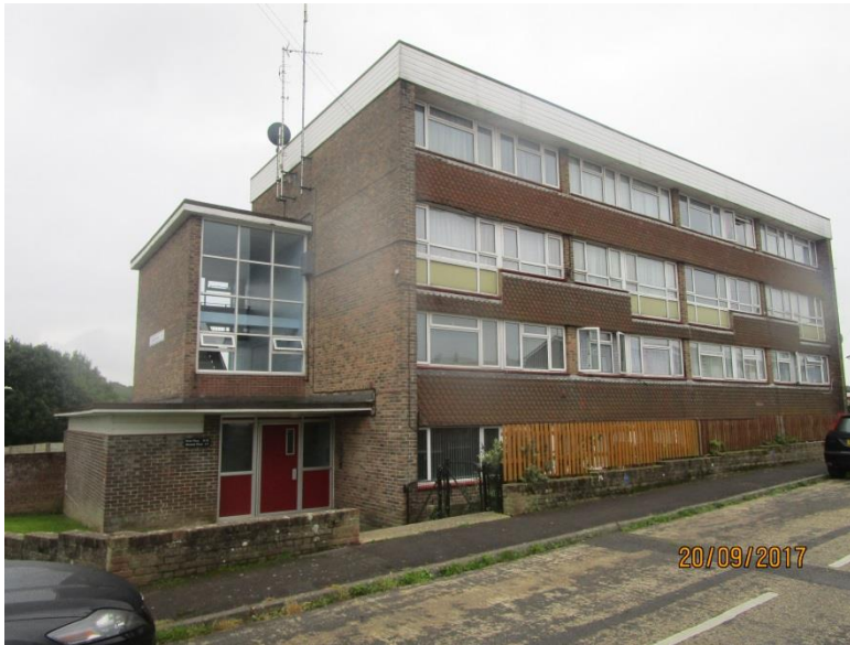
Photo 1 - Front Elevation showing boundary fencing
