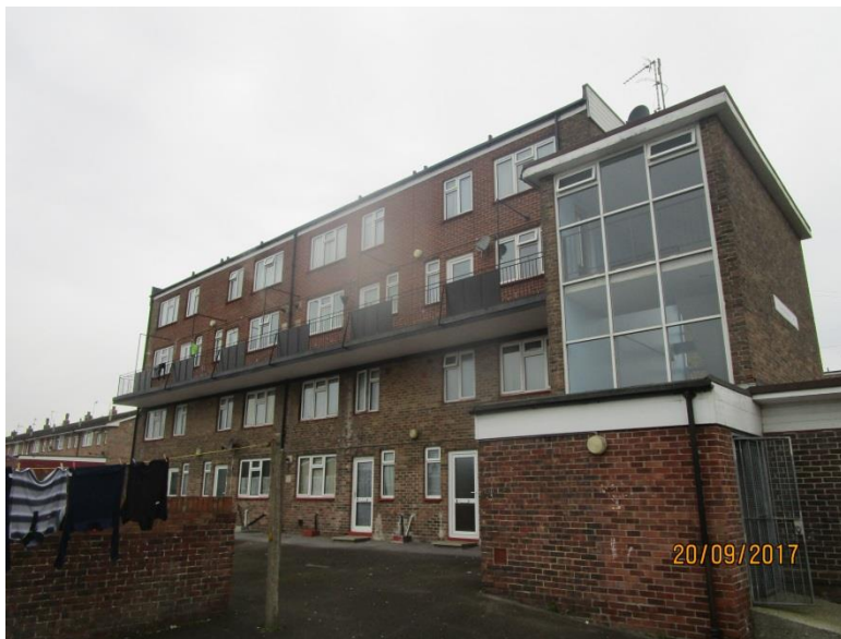
Photo 2 - Rear elevation showing balcony walkway
