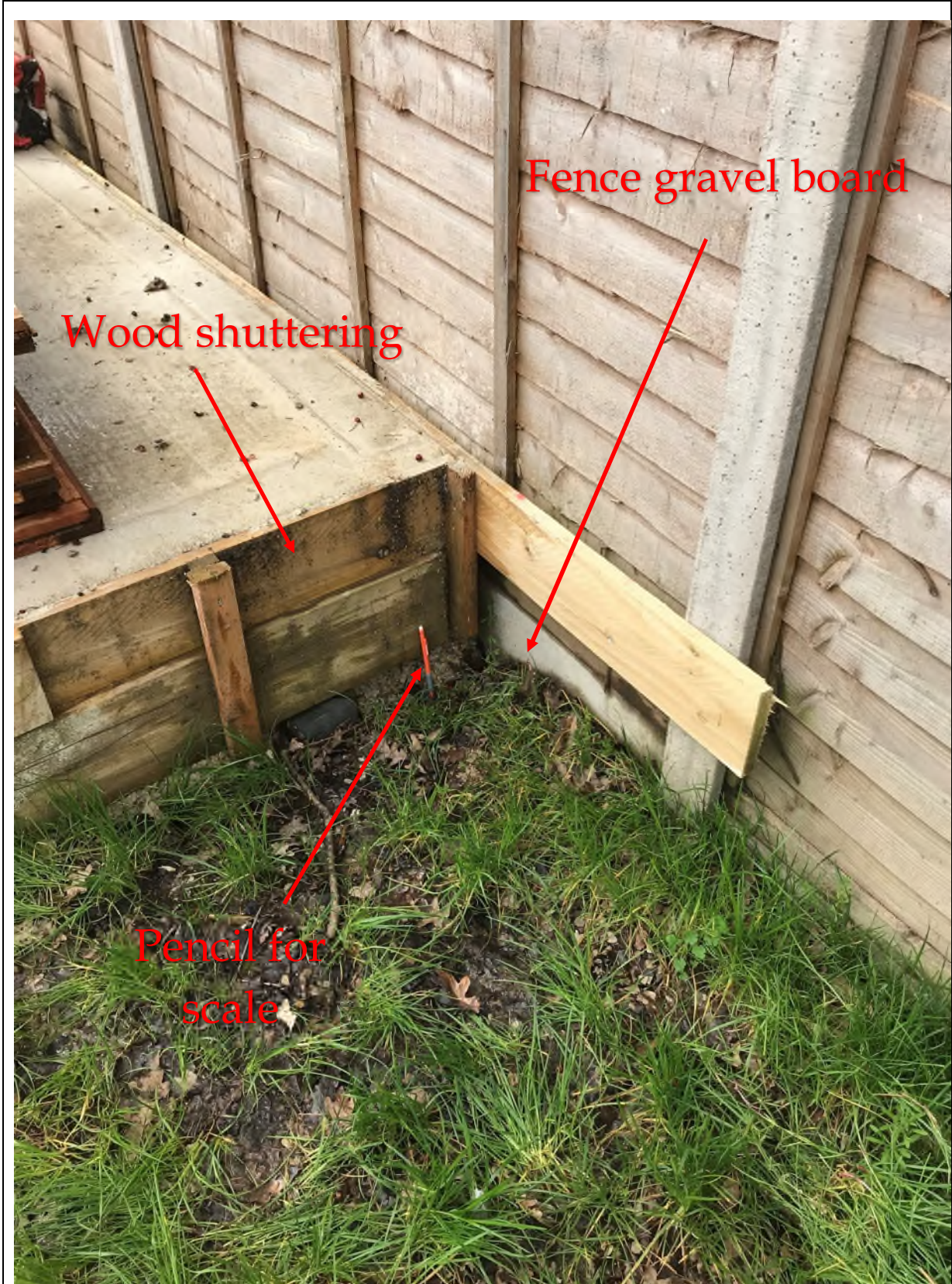
Photo 4: Concrete base showing wood shuttering and relationship with rear boundary fence
