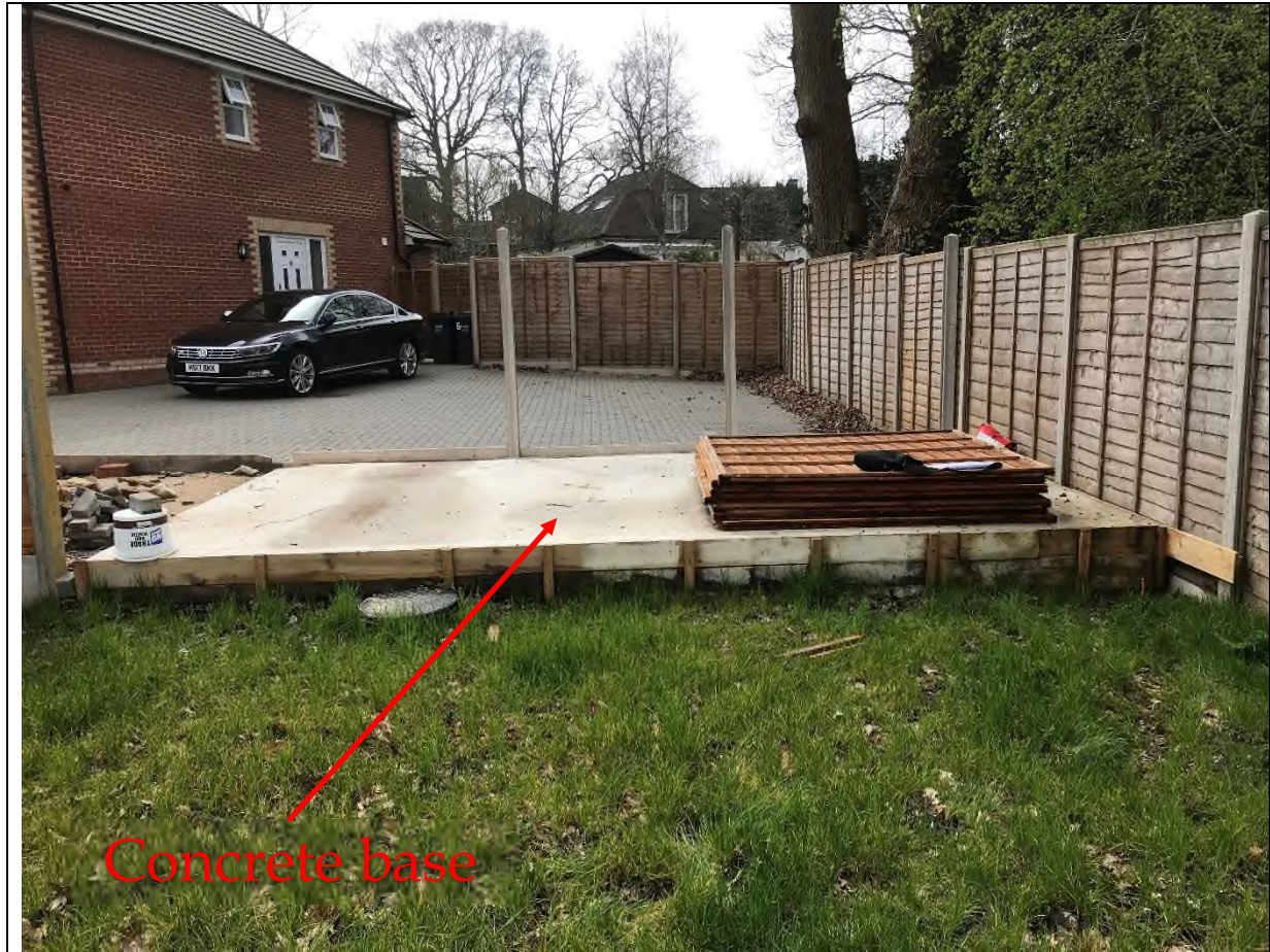
Photo 3: Concrete base from north east side of site looking south west
