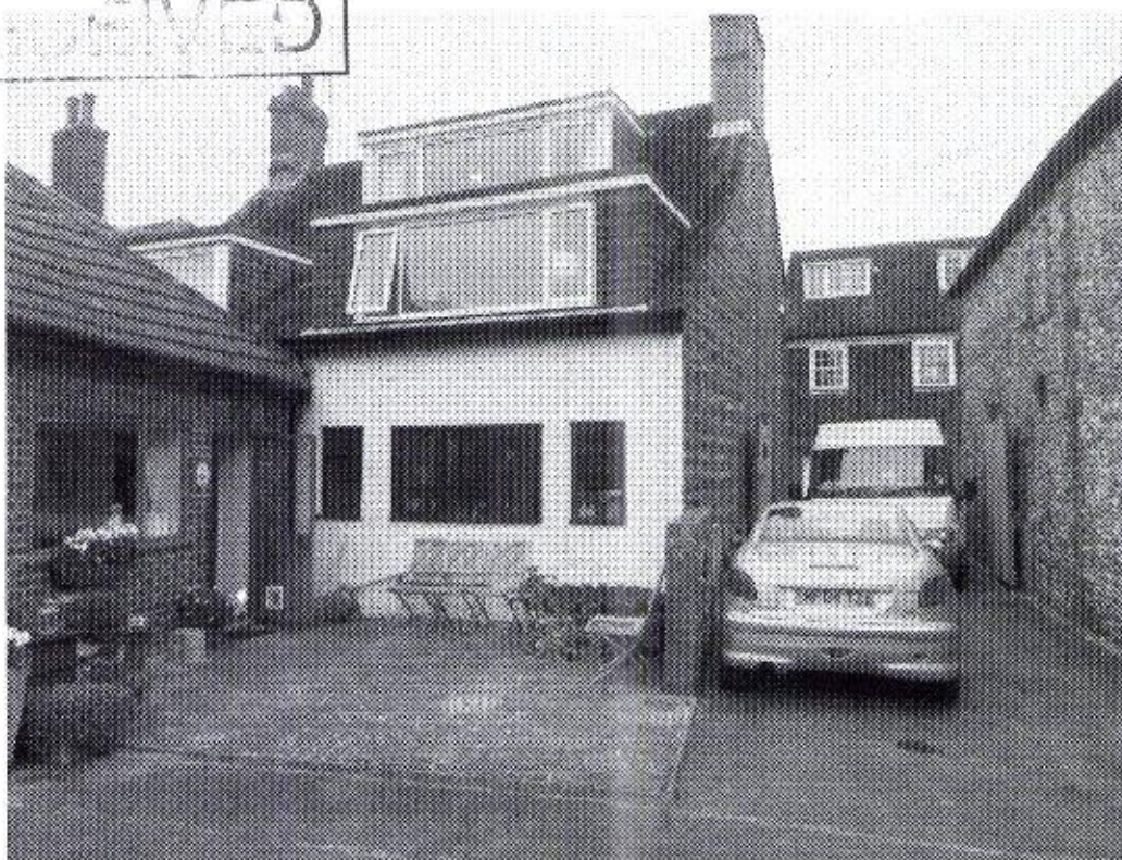
Rear view of 15 King Street.
