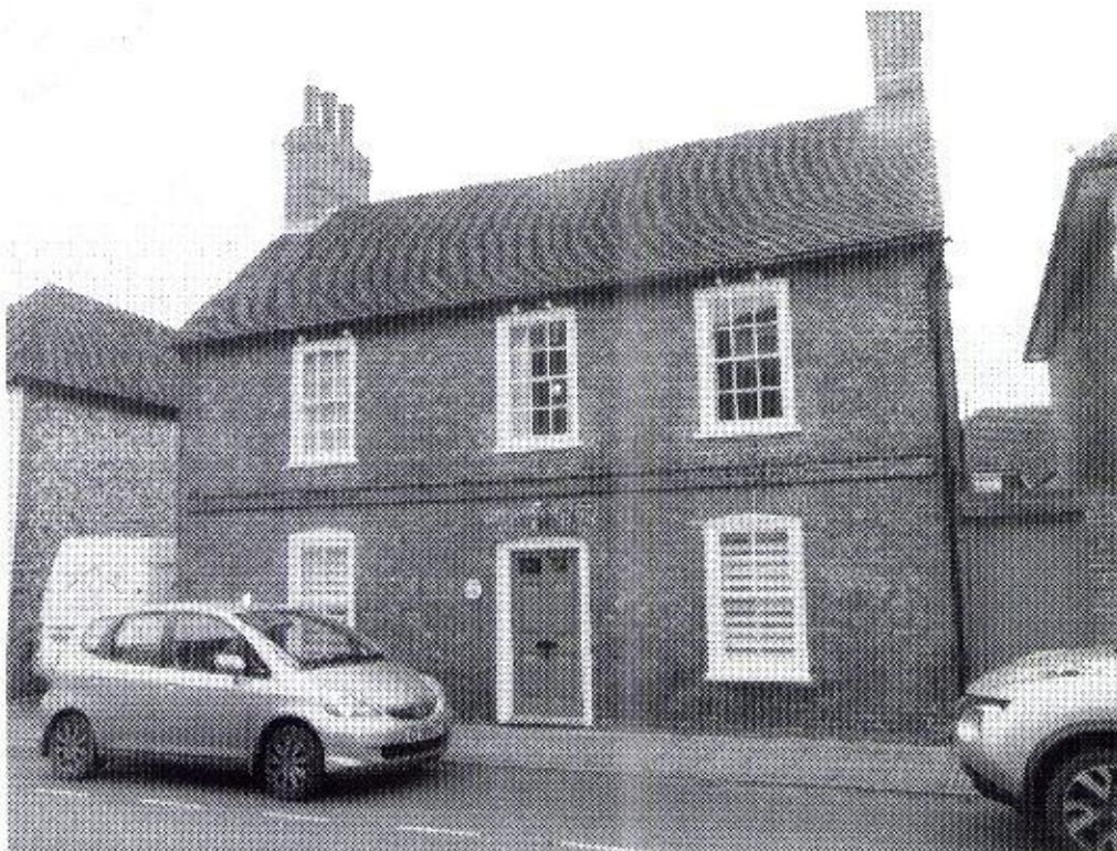
Road view of 15 King Street.
