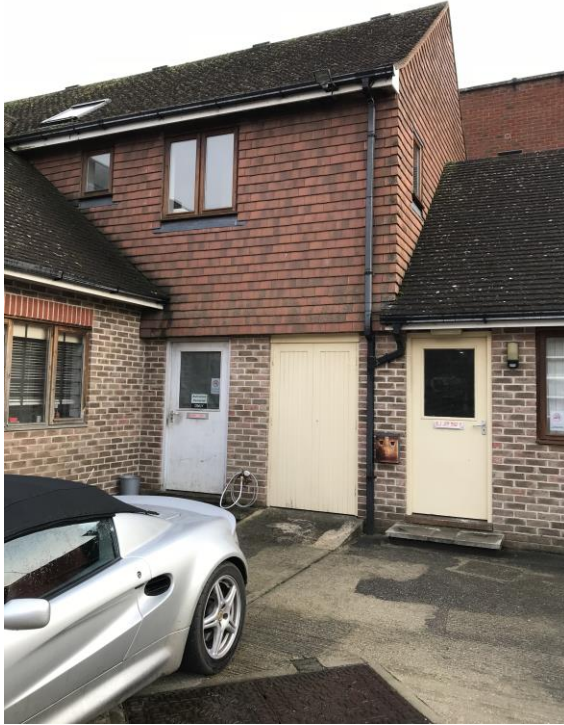
Access to Units 14 and 15 where proposed porch will be placed
