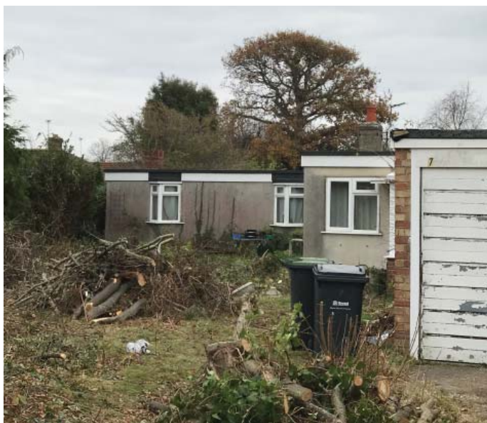
Existing dwelling at 7 Selsmore Avenue
