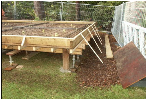
Photo 34: Small diameter piles (less than 150mm) are an effective means of supporting structures in RPAs with minimal disturbance.
