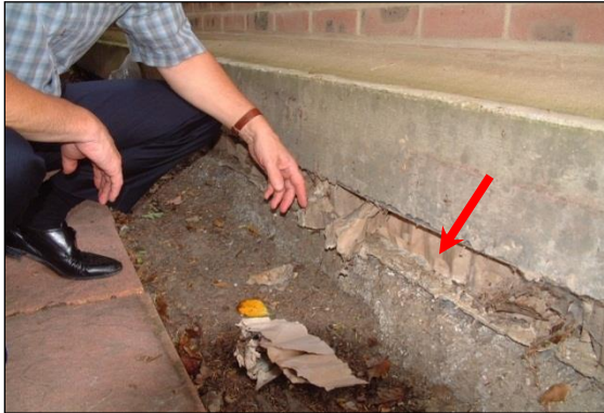
Photo 40: Where a slab is cast on site, a biodegradable void-former (red arrow) temporarily supports the weight of the liquid concrete until it sets. The void-former can then be wetted and washed away to leave a void or left to degrade naturally, both of which allow movement of air beneath the slab.
