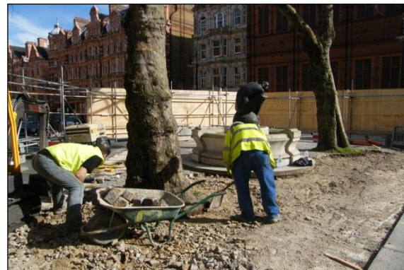
Photo 21: These trees had impermeable surfacing right up to their trunks, which had to be removed by hand before installing new structures.
