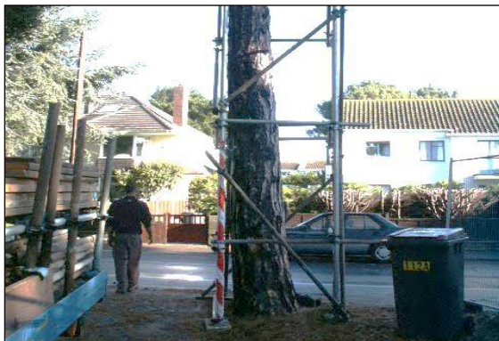
Photo 4: A scaffold braced framework surrounding the trunk reduces the risk of accidental impact.
