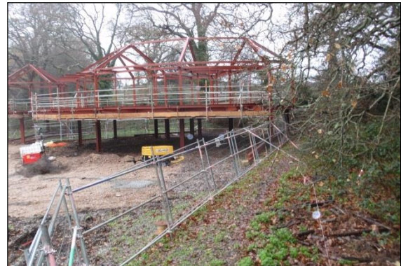
Photo 35: It is possible to support very large structures on piles within sensitive RPAs without any significant adverse impact on tree roots.
