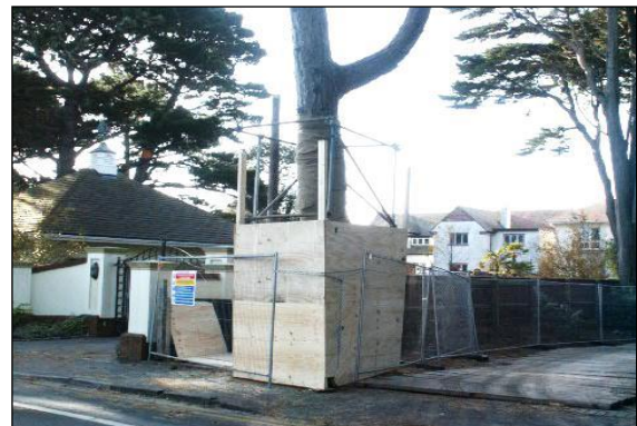
Photo 5: Board secured to scaffold framework adds another layer of protection for vulnerable trunks and branches.
