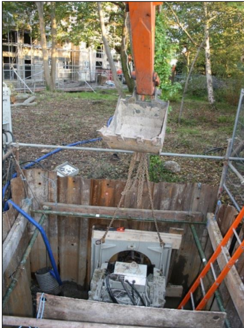
Photo 42: If possible, thrust boring is the preferred option for installing service routes through the RPAs of important trees, but there has to be space at the start and finish to dig substantial working pits.
