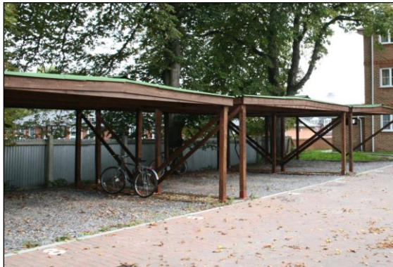
Photo 32: These carports are formed by wooden posts above a three dimensional cellular no-dig and load-spreading surface of permeable crushed stone.
