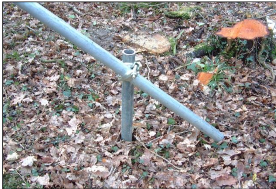
Photo 2: Close up of bracing detail, essential for increasing the stability of the vertical framework.
