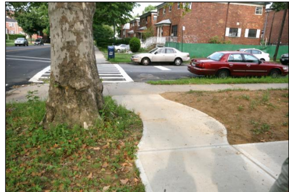
Photo 27: In some situations, it may be appropriate to cast a free floating concrete surface directly onto the soil surface provided provision is made to prevent soil contamination while the concrete is being poured, i.e. an impermeable membrane separating the concrete from the soil.
