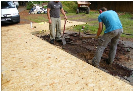
Photo 14: Careful hand-digging using conventional tools is acceptable for exposing roots in RPAs.
