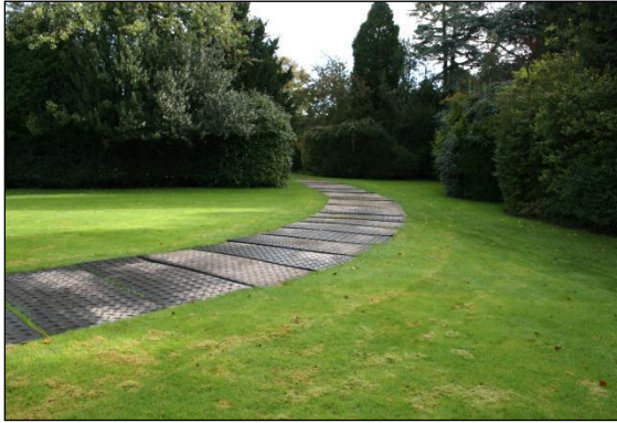
Photo 18: Ground protection must be used where repeated foot or vehicle traffic could cause compaction in sensitive RPAs. It can be as simple as plywood for pedestrians, but must be more robust for vehicles.
