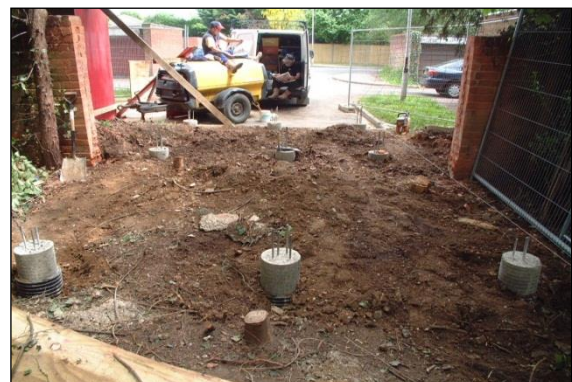
Photo 39: Piles can also be used to support bridges across sensitive RPAs, but the temporary ground protection has to be removed before the main structure is either imported in or cast on site.
