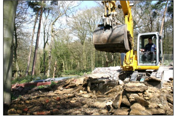
Photo 19: Machines with a long reach can be used to lift out heavy surfacing and structures as long as the machine sits outside the RPA and the exposed surface is protected before there is any further access.
