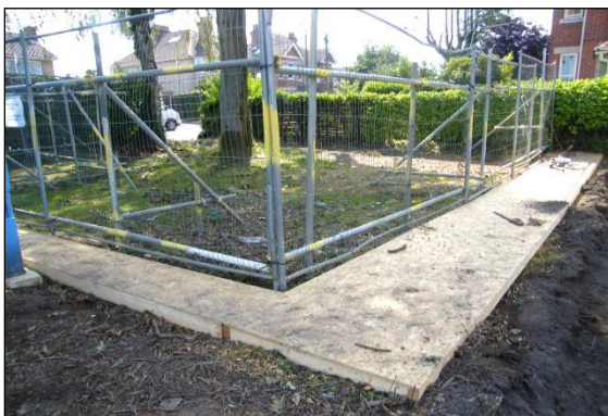
Photo 8: Plywood fixed to a wood frame is another effective method of protecting soil from pedestrian compaction.
