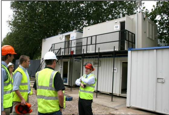
Photo 12: A combination of retaining existing surfacing and using temporary construction cabin accommodation can be a very effective means of preventing damage to sensitive areas.
