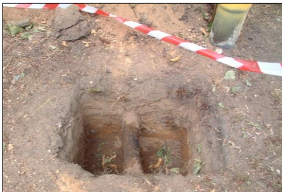
Photo 36: Where piles are proposed close to trunks, it is essential to excavate 50–75cm deep to see if there are any significant roots in the way, with provision to move the pile location if roots are found (note the pile was finally installed to avoid this root).
