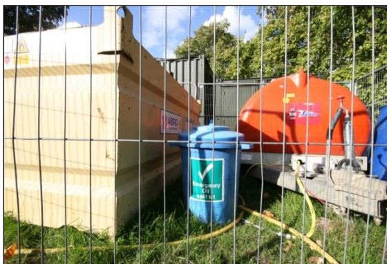
Photo 44: Where fuel or other chemical are stored on site, it is now standard practice to have emergency spillage kits available to restrict the environmental impact of accidents.
