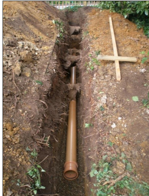
Photo 43: Continuous trenches dug by hand so that important roots can be retained (with the service ducting threaded beneath) is an effective means of minimising damage (note the ground protection boards with soil piled on top on the left).
