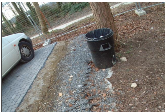
Photo 24: A conventional concrete haunching can be used to retain new surfacing as long as it is not dug into a trench - here it is placed on top of the CellWeb layer.
