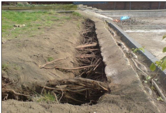
Photo 16: Air spades are particularly useful where roots are very dense.
