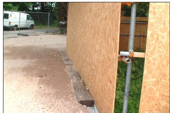
Photo 25: Although this is only a temporary surface, railway sleepers pinned into the ground can be used to retain the edges of new surfacing.
