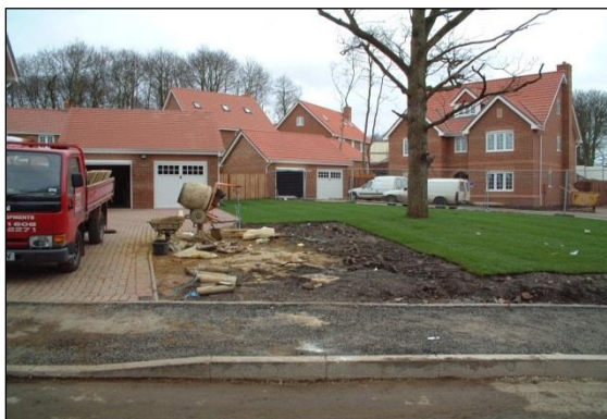
Photo 46: The RPA of this tree was not effectively protected during construction and excessive compaction of the soil meant it died soon after this turf covered up the damage.
