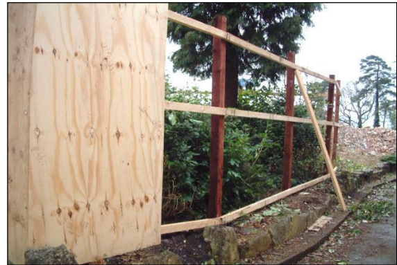
Photo 3: Board specification on secure wooden posts is a suitable alternative to the standard braced scaffold design.
