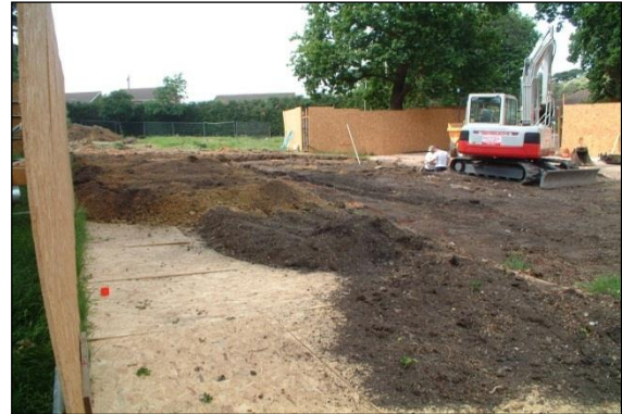
Photo 7: Spreading soil excavated from footings is an effective way of buffering the plywood surface from the wear of light vehicles.
