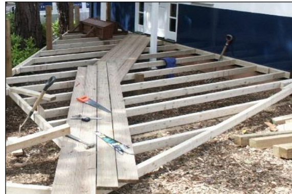
Photo 33: This deck supported above the ground on small posts provides a low-impact alternative to conventional stone patio surfacing in RPAs.
