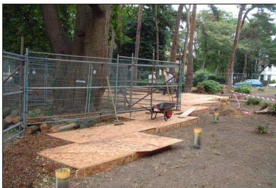
Photo 38: Once the piles have been installed (yellow tops), the ground protection to support the piling rig is removed ready to fix the void-former onto the bare soil, in advance of pouring the building slab.
