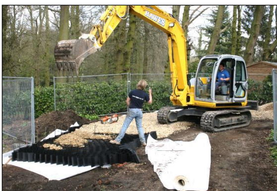
Photo 10: Cellular products are a very effective means of providing ground protection where heavy vehicle use is expected. Here, it is being used to temporarily widen an existing road, to be removed once the construction is finished.
