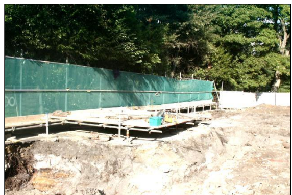
Photo 9: A scaffold framework attached to the main scaffold fencing can be used to support either scaffold planks or plywood to create an elevated platform with a gap beneath.
