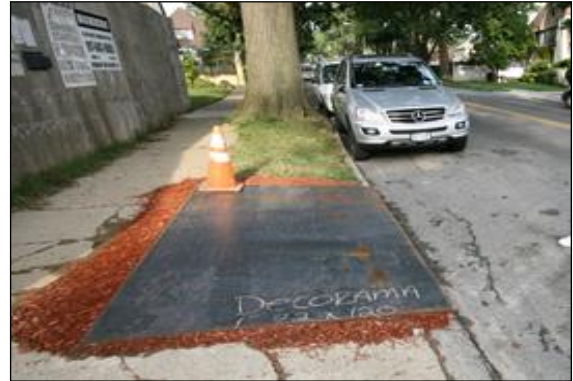
Photo 13: Steel plates can be an effective way of temporarily reinforcing weak surfacing over a construction access during the development activity.
