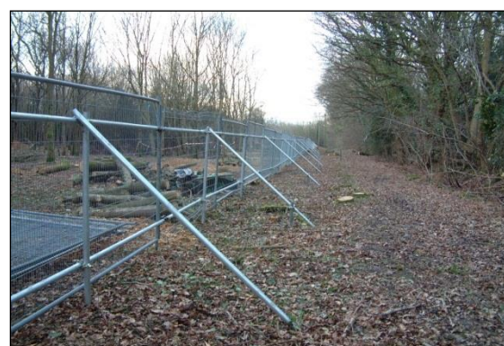
Photo 1: Heras fencing wired to scaffold braced posts is a robust and effective interpretation of the BS specification.
