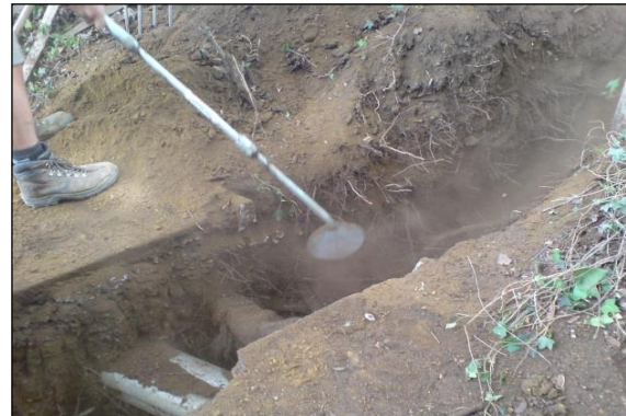
Photo 15: Air spades are very effective at exposing roots and services with minimal damage.
