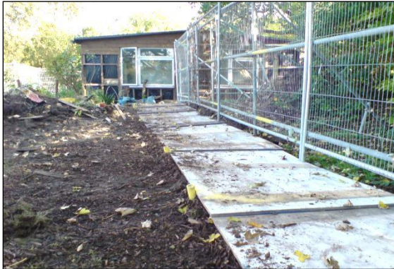
Photo 6: Heavy-duty plywood set onto a compressible woodchip layer and pinned into position is suitable to spread the loading from pedestrian access.
