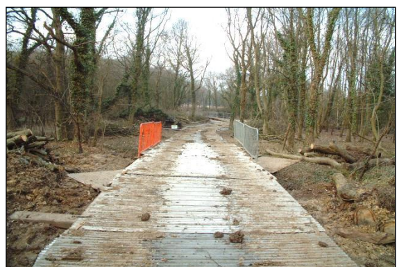
Photo 11: Custom designed sectional tracks can be joined to support very heavy traffic use through sensitive areas.
