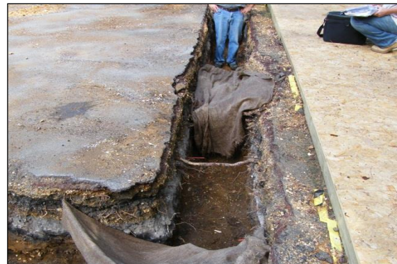
Photo 17: Exposed roots must be protected from light, drying out and extremes of temperature by covering with hessian sacking and boards until they can be covered back with soil.
