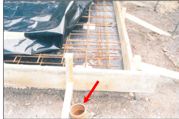
Photo 41: This reinforced base slab for a double garage has drainage provision (red arrow) beneath the structure to redirect roof runoff to supply roots with water.
