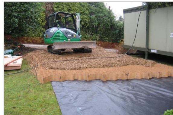
Photo 23: The stone-filled cells spread the load of traffic and the geotextile membrane on the ground prevents migration of the stone into the soil profile.
