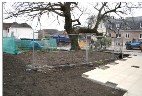
Photo 47: This tree had tarmac parking within its RPA that was removed and replaced with an organic mulch near the trunk and limited no-dig surfacing on the outer edges of its RPA.
