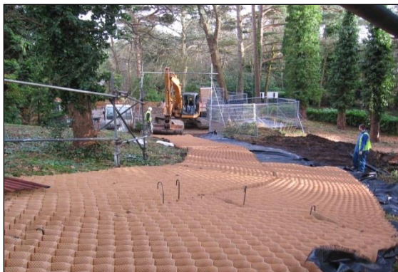
Photo 22: The three-dimensional cells are opened up, spread across the area to be surfaced and pinned in place ready for the stone filling.
