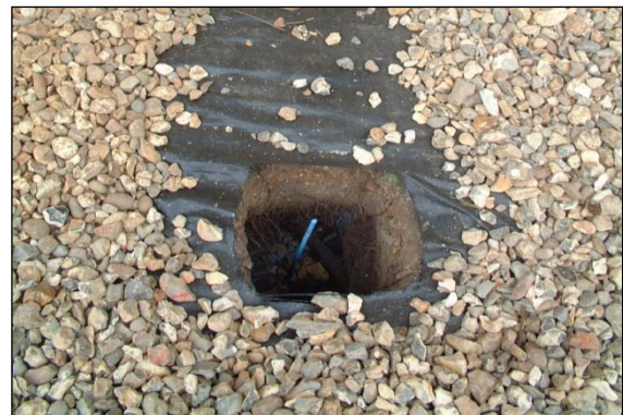
Photo 37: Ground protection must be used to spread the load of the piling rig once excavation has confirmed that no substantial roots are in the preferred pile location.
