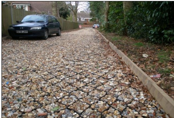
Photo 26: Wooden board pinned in place or held in position with backfilled topsoil can provide more informal and rustic surface edging.
