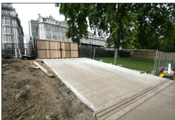
Photo 28: This temporary access for heavy construction traffic on the outer edge of a RPA is a concrete slab cast above ground level and will be removed when the project is completed.
