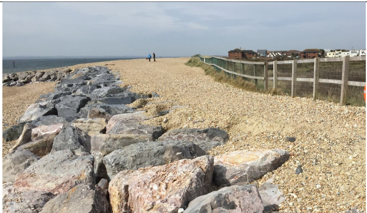
Photo 1.3 The completed rock revetment at the Eastoke Point Scheme
