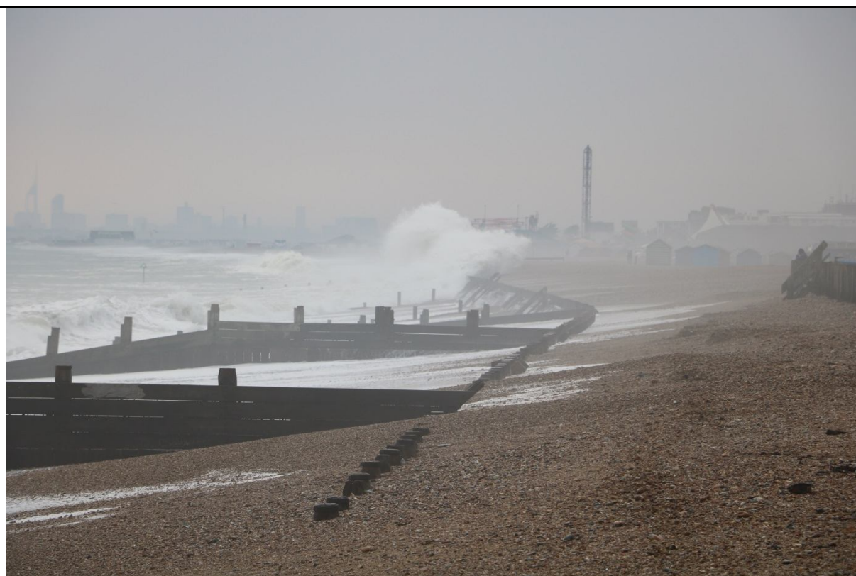
Photo 1.1 Hayling beach during a significant swell period in December 2016
