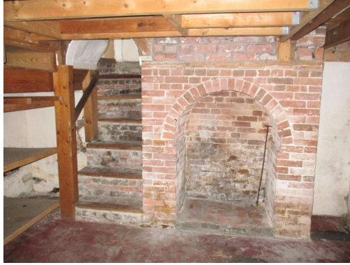
Fig 5: Cellar showing raised floor above
