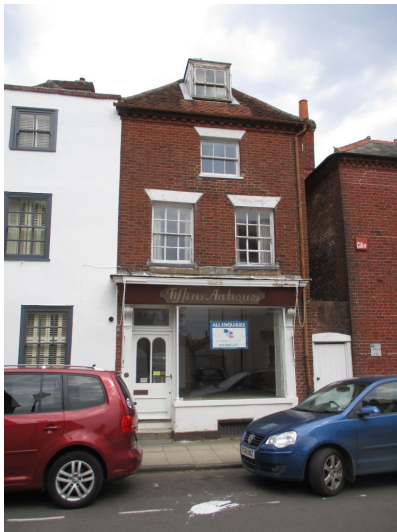
Fig 1 – Front view of property from Queens Street
