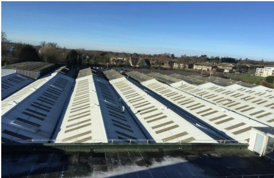
Plate 6: Corrugated metal roof with composite skylights of the main factory building
