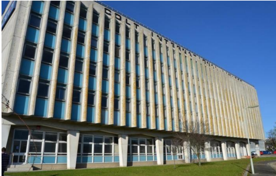
Plate 7: Front (eastern) elevation of Building 1 constructed from concrete with a flat roof
