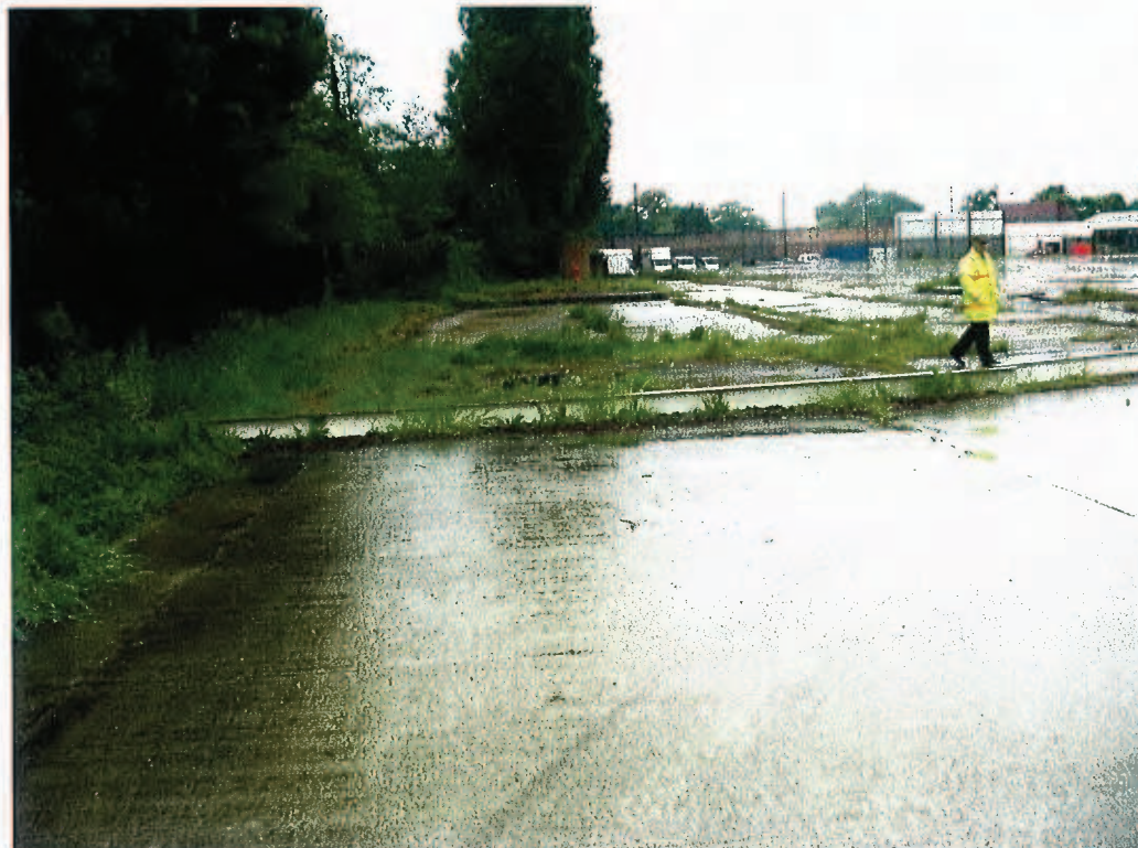
PHOTO 6 - Former location of excavated underground oil storage tank.
