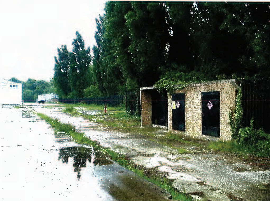
PHOTO 8 - Former solvent and petroleum store adjacent to demolished Scalextric factory.
