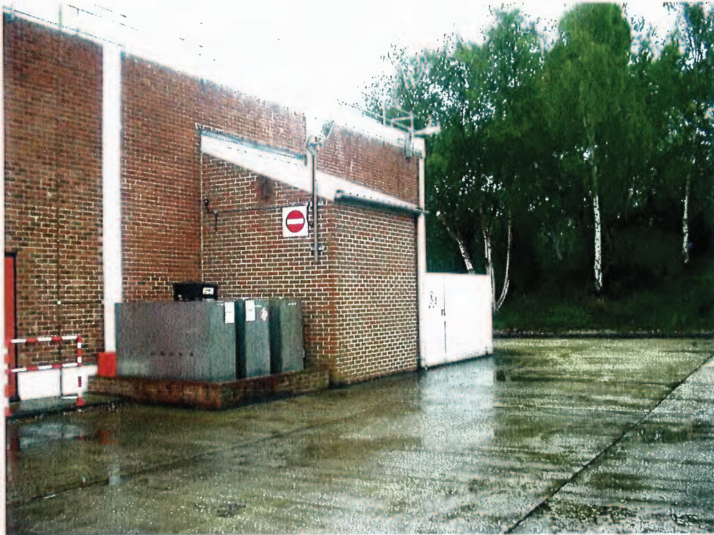
PHOTO 1 - Waste oil tanks, with small bund.
