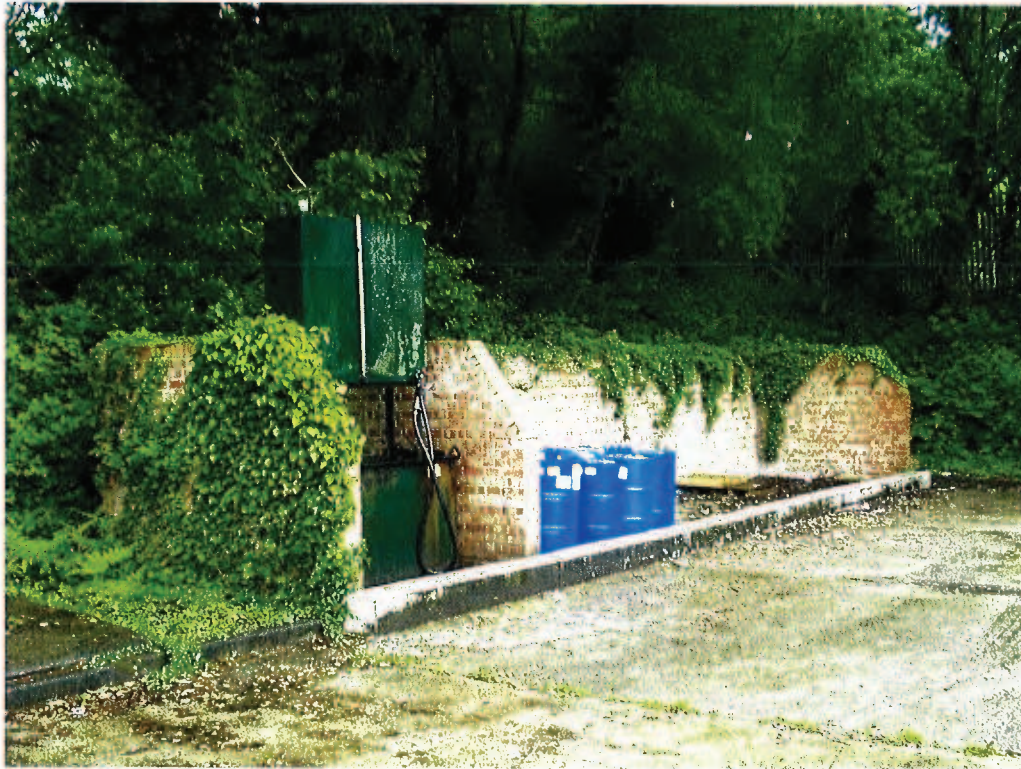
PHOTO 3 - Diesel dispensing pump and banded chemical drum storage.
