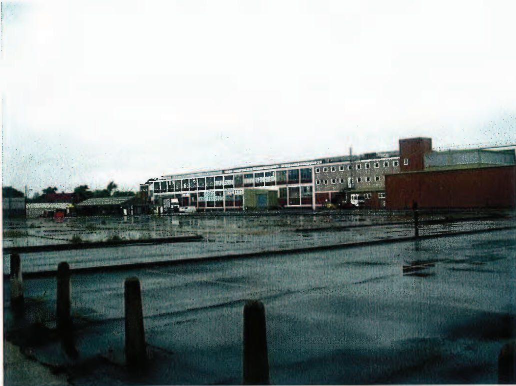
PHOTO 5 - Area of former Scalextric Factory.
