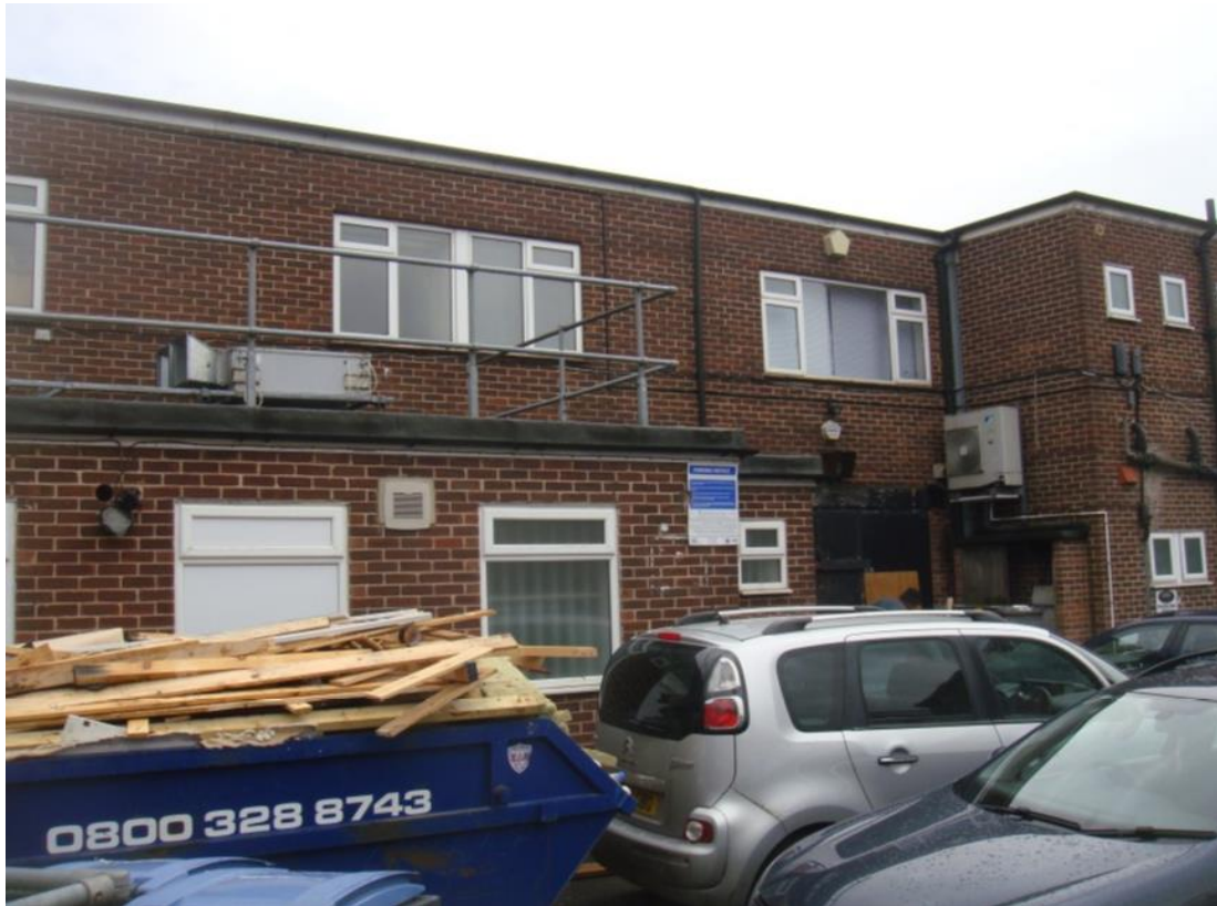
Image 2: Rear elevation of the site and surrounding units
