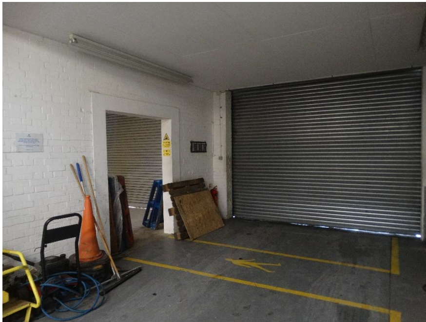
Photo 4 – showing the inside of the delivery doors to unit 2 (and link to unit 3).
