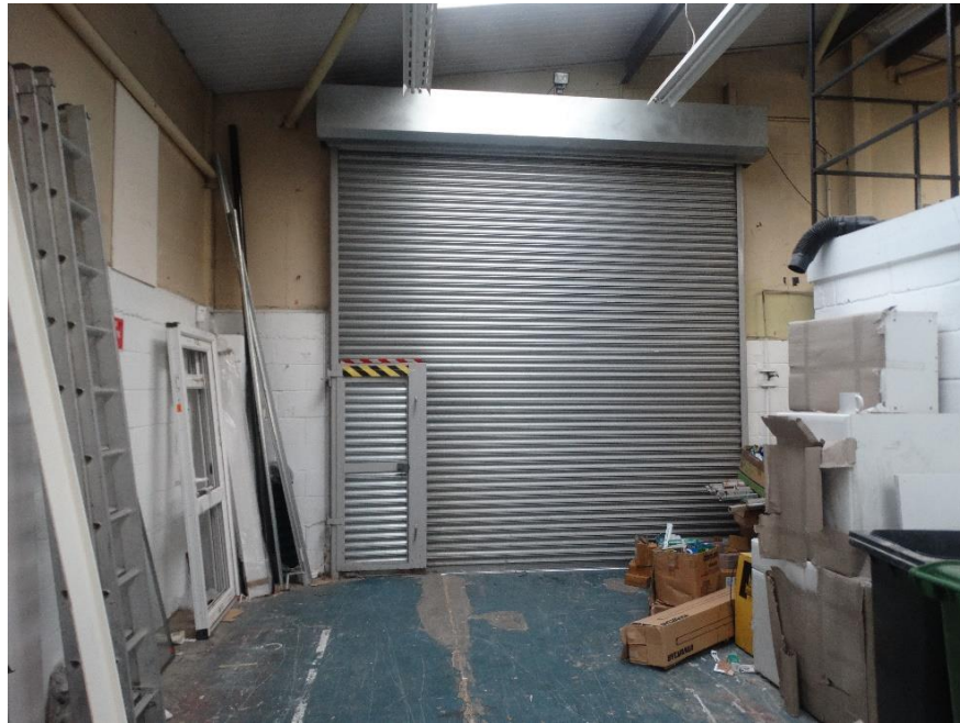
Photo 3– showing the inside of the delivery doors to unit 1
