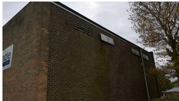
Plate 4.2: Brickwork in Good Condition
