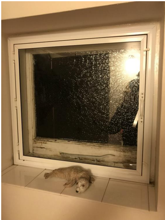
Figure 7: Internal view of window C
