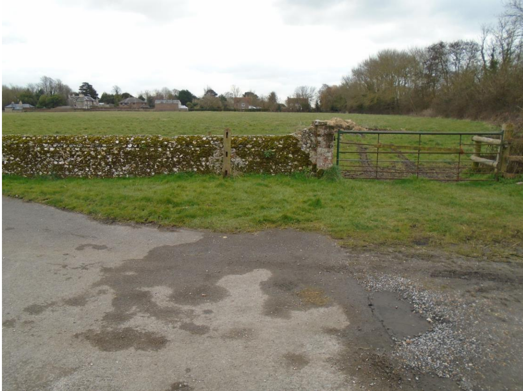
Figure 12. Low flint wall (No.7)
