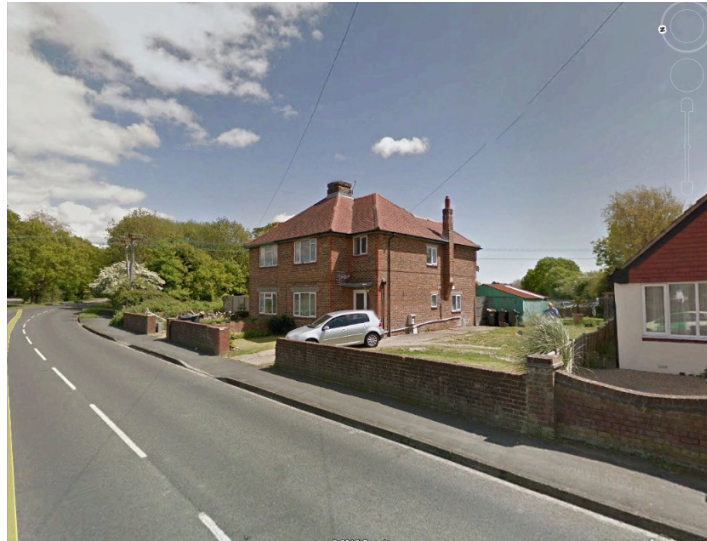
Fig1 View of site looking north east
