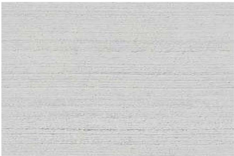
Concrete to forecourt
