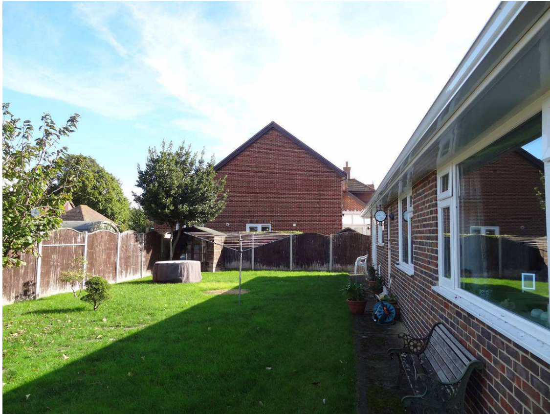
Photo 1 –View of the rear and garden looking east. Adjoining house at No.11b seen beyond.
