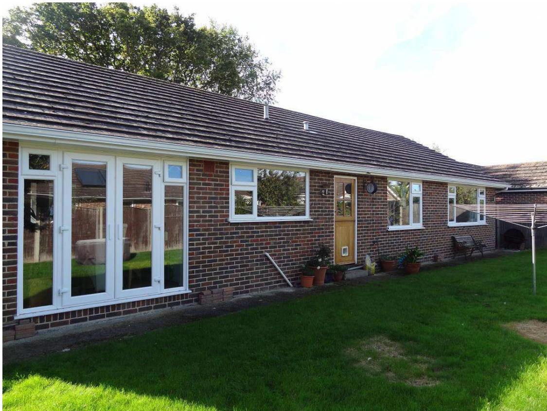
Photo 2 – View of rear elevation looking south-west..
