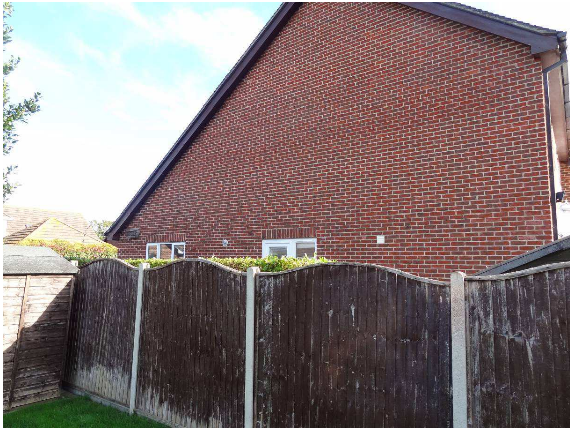
Photo 5 – View from rear garden towards west flank wall of 11b Salterns Lane.
