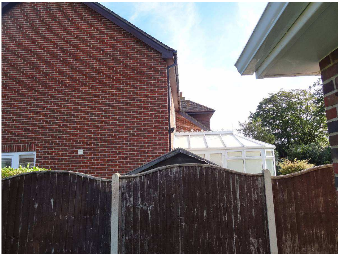
Photo 6 – View from rear garden towards west flank and front of 11b Salterns Lane.
