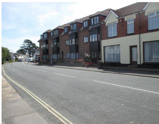
Photograph 4: Station Road Pedestrian Environment
