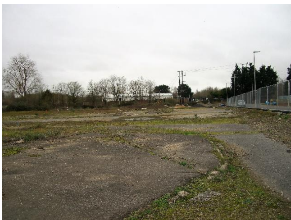
Photograph 5 – view to west & hardstanding
