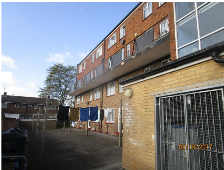
Photo 2 - Rear elevation showing balcony walkway
