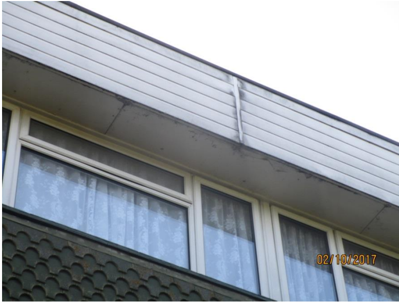
Photo 3 - Existing Fascia Board and Soffit
