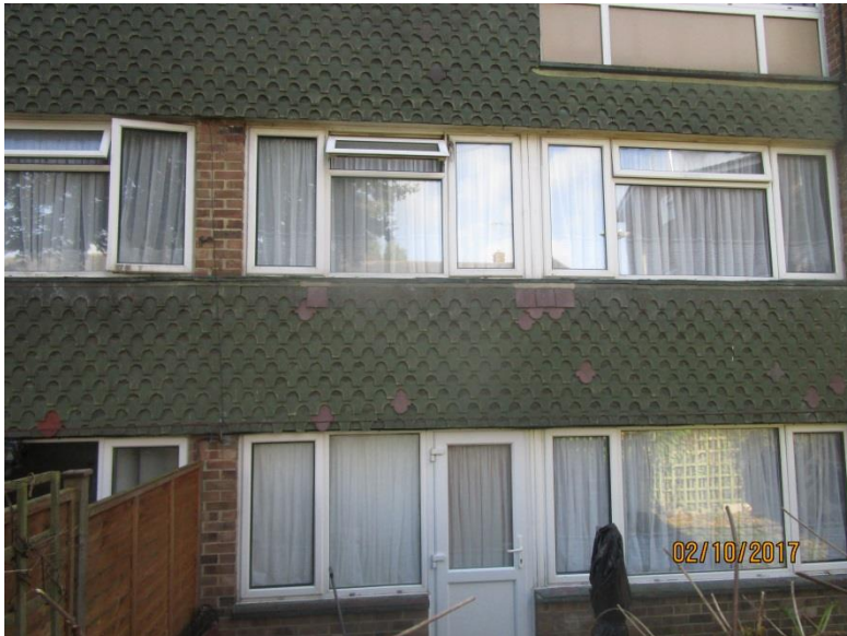
Photo 4 - Tile hanging to front elevation
