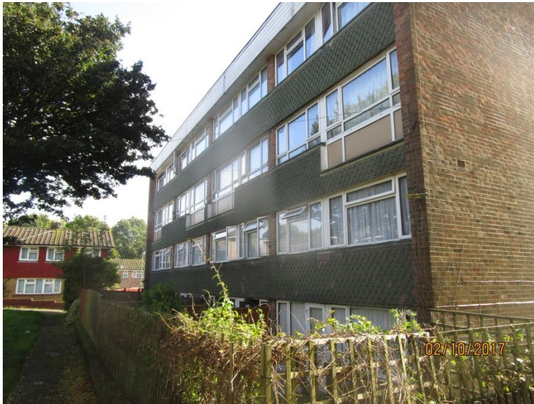
Photo 1 - Front Elevation showing boundary fencing
