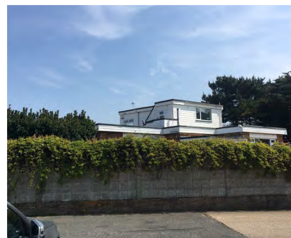
Boundary wall and hedge screen to Sparkes Carpark
