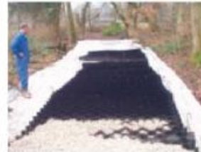
Installation of the CellWeb™ system.
